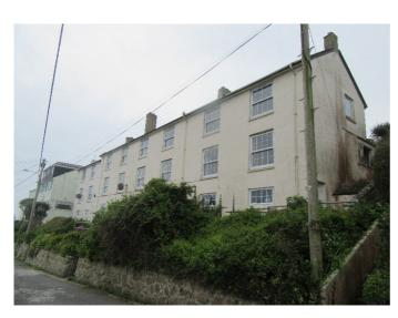
**Description:** The properties included within this application are two blocks; 32-34 and 36-42. The properties are served over 3 floors and comprise of solid rendered external walls with PVCu sash windows and PVCu glazed doors. Concrete canopies are provided above the doors with a slate roof to the blocks.
