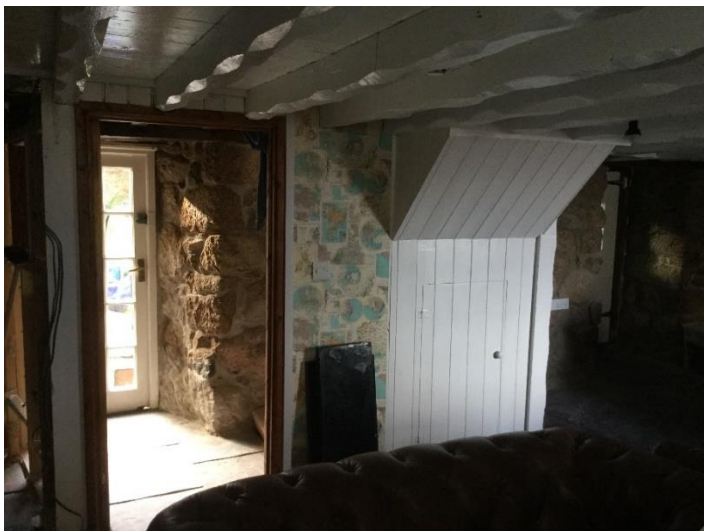
Ground floor – modern staircase partitions and cladding
