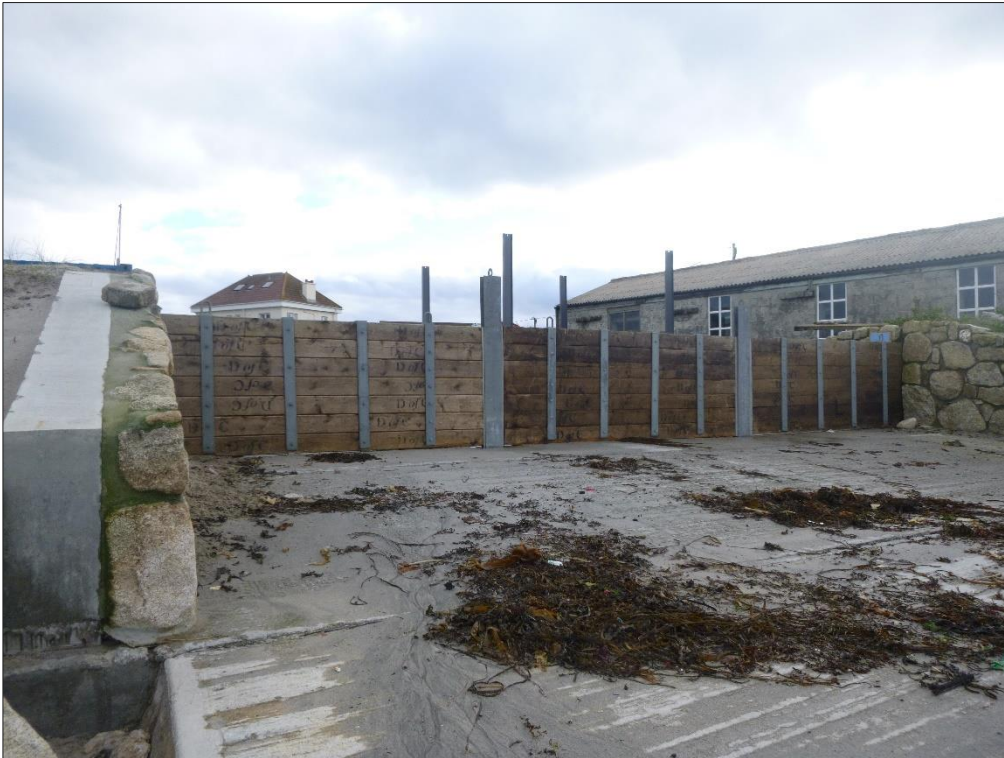
Figure 6: Boatyard slipway protected by stop-logs at the southern end of the beach. Logs branded with D of C (Duchy of Cornwall) who are believed to be responsible for slipway and existing dune defence.
