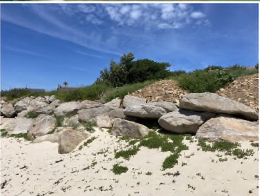
3 SITE 2 & 3b. Great Porth section showing ad hoc rock placement
