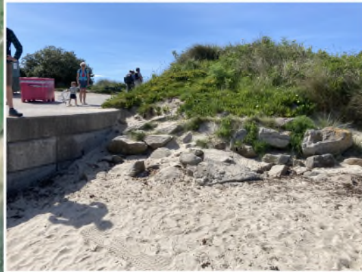
8 SITE 8. Quay eroded section
