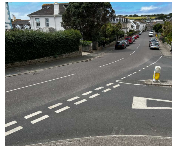
Very wide junction mouth combines with poor visibility from opposite footway and high approach speeds to create a hazardous environment.
