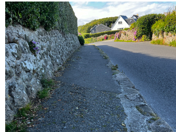
Footways are in poor repair and their kerbs are a fall hazard
