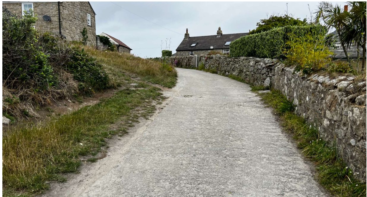
Typical off-island concrete road
