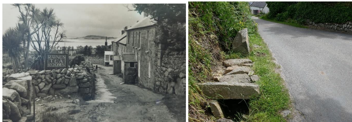
Fig 124 St Martin's and St Mary's: Traditional stone-built drains or 'bolts' (left to right).
