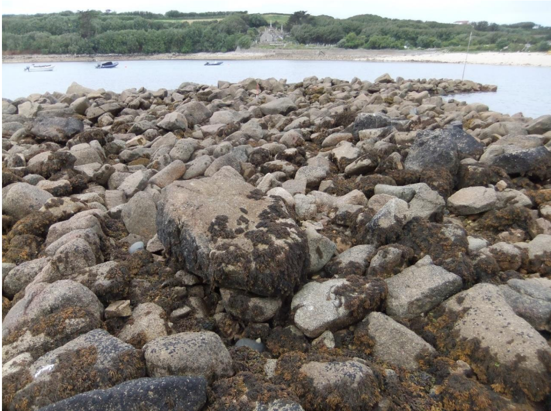
Fig 34 St Mary's: Old Town's south pier, with its inner face curving out from front left (past 1m scale in middle ground in front of the church) and displaced stones to right.
