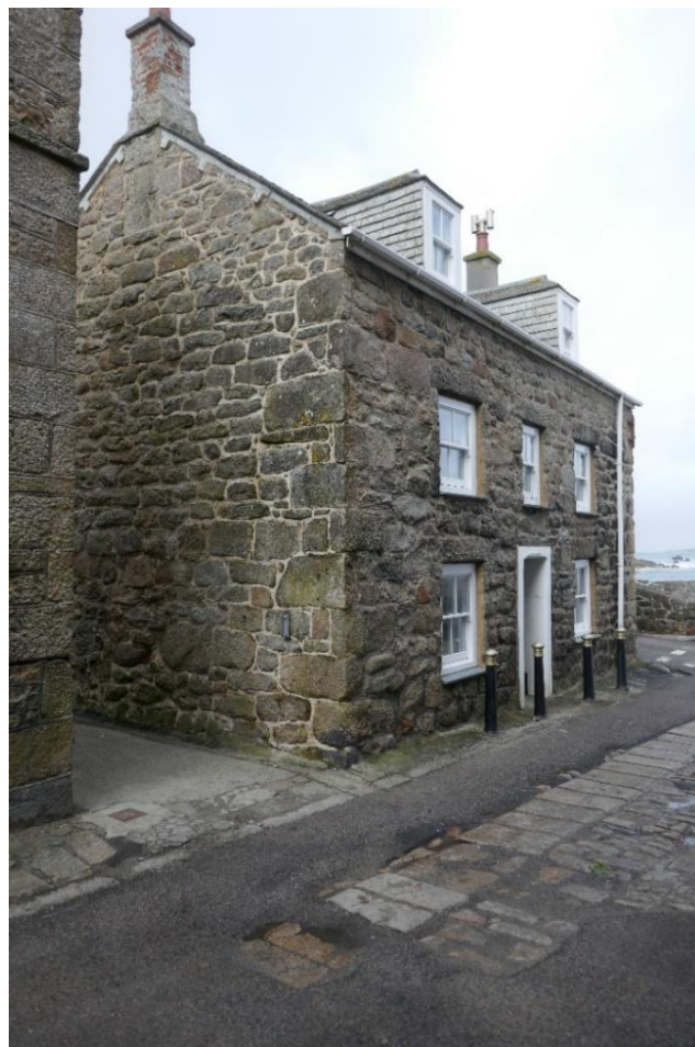
Fig 58 St Mary's: Quay House, Quay Street, early house near the head of the Elizabethan quay, with previous roofline visible in its gable wall.
