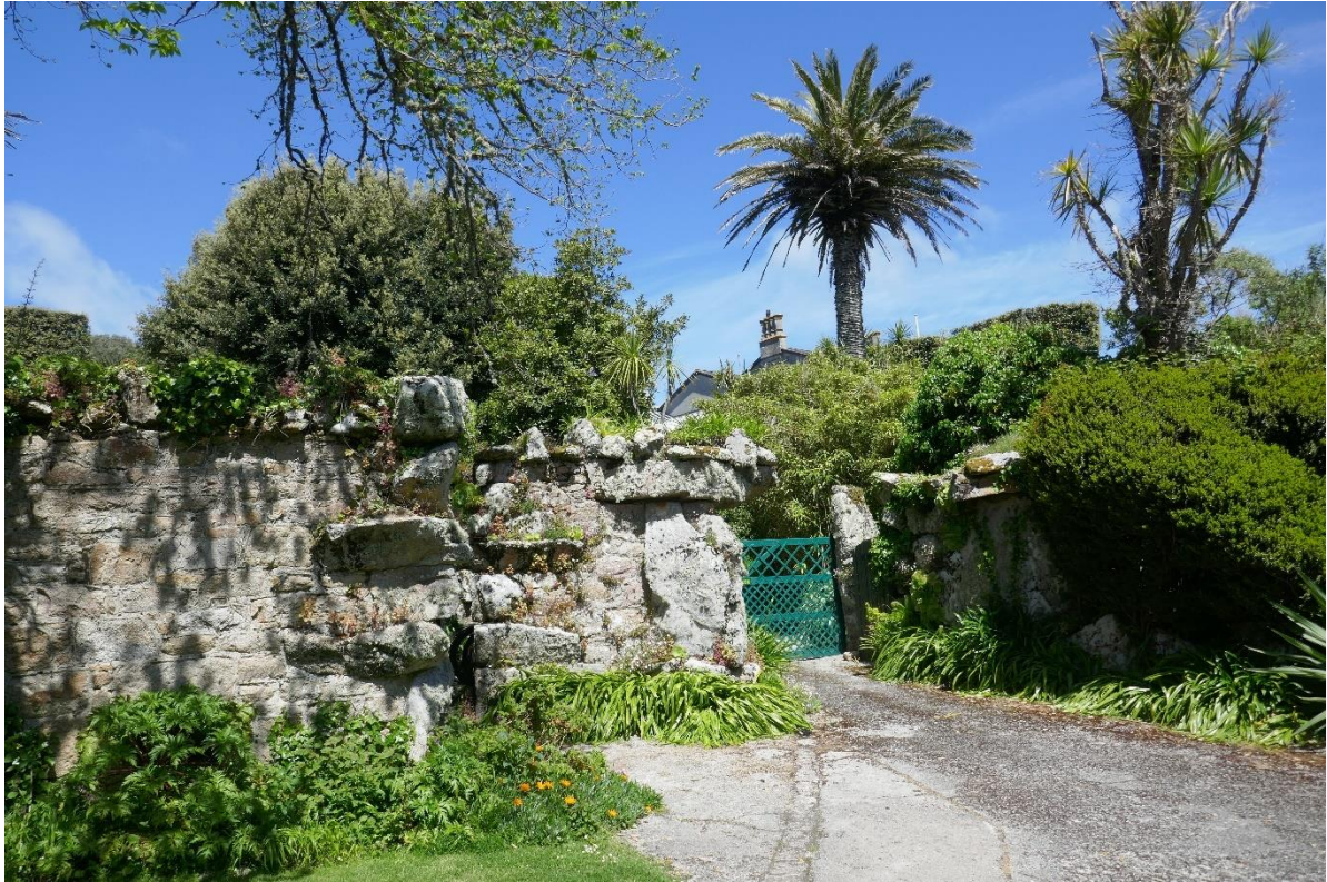
Fig 134 Tresco: Entrance to inner grounds of Tresco Abbey with boulder style walling. The wall design here shows a hierarchy in the application of this estate style; being on the inner approach to the mansion, it has boulders set in several tiers as well as on top.
