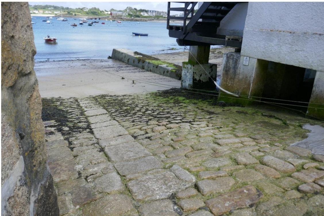
Fig 87 St Mary's: Atlantic Slip (named after a pilot cutter formerly based here), the old Custom House Slip, with with paved wheel courses like those of west Quay Street.
