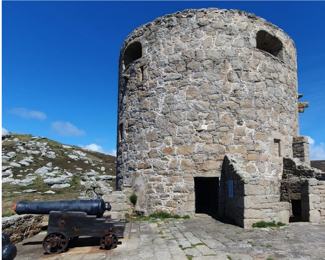
Fig 49 Tresco: Cromwell's Castle, an unusual design, with round tower and protruding granites built into it possibly to create the impression of guns when seen in profile.
