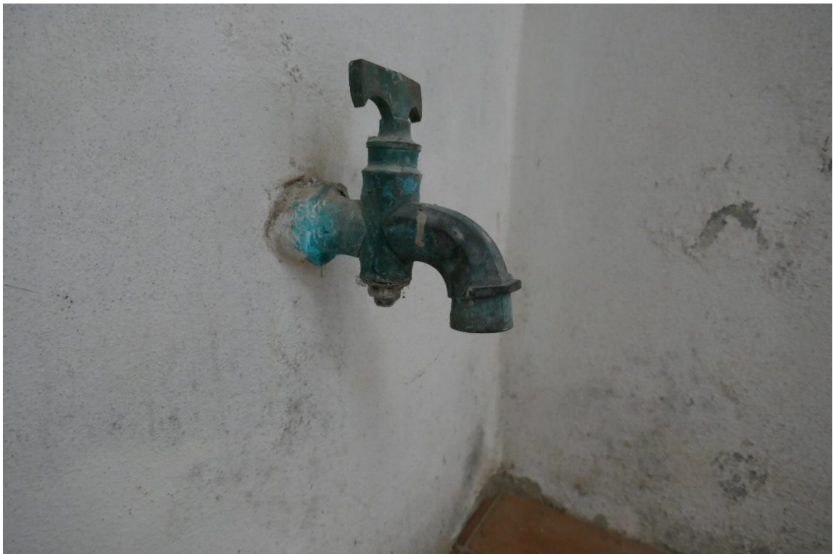
Fig 161 St Mary's: Original tap to wall of integral water tank, in Altamira, Porth Loo. These features show design of houses to harvest rainwater continued over 200 years.
