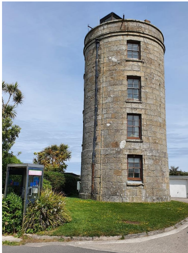
Fig 91 St Mary's: Telegraph Tower, built as a semaphore tower superseding St Martin's flag signal station. The semaphore gear with moveable arms stood on its roof.
