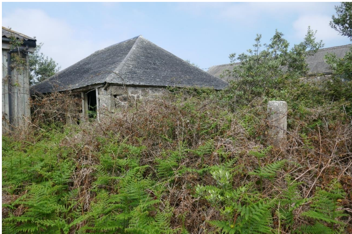
Fig 154 St Mary's: Hipped scantle roof giving an almost pyramidal effect to a squarish building of c1890 at Content, designed as a bull pen (James Sherris pers. comm.).
