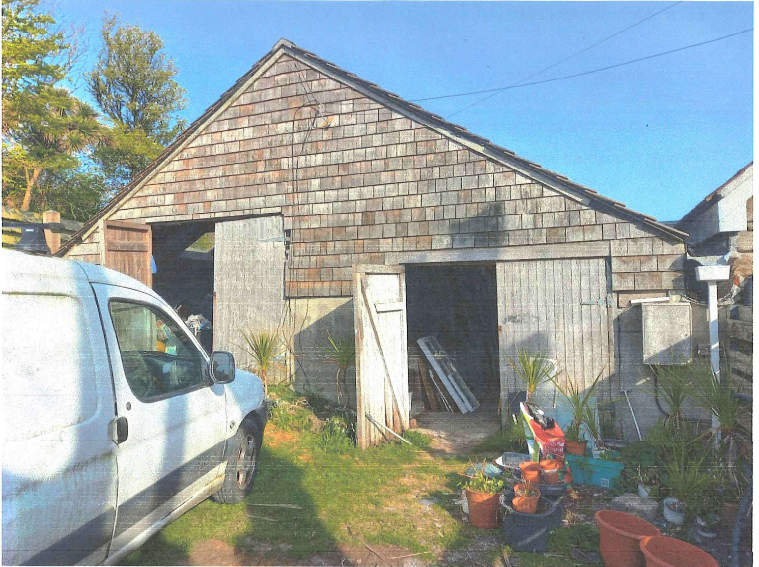
Photo 1. Castle Farm Workshop south-east elevation
