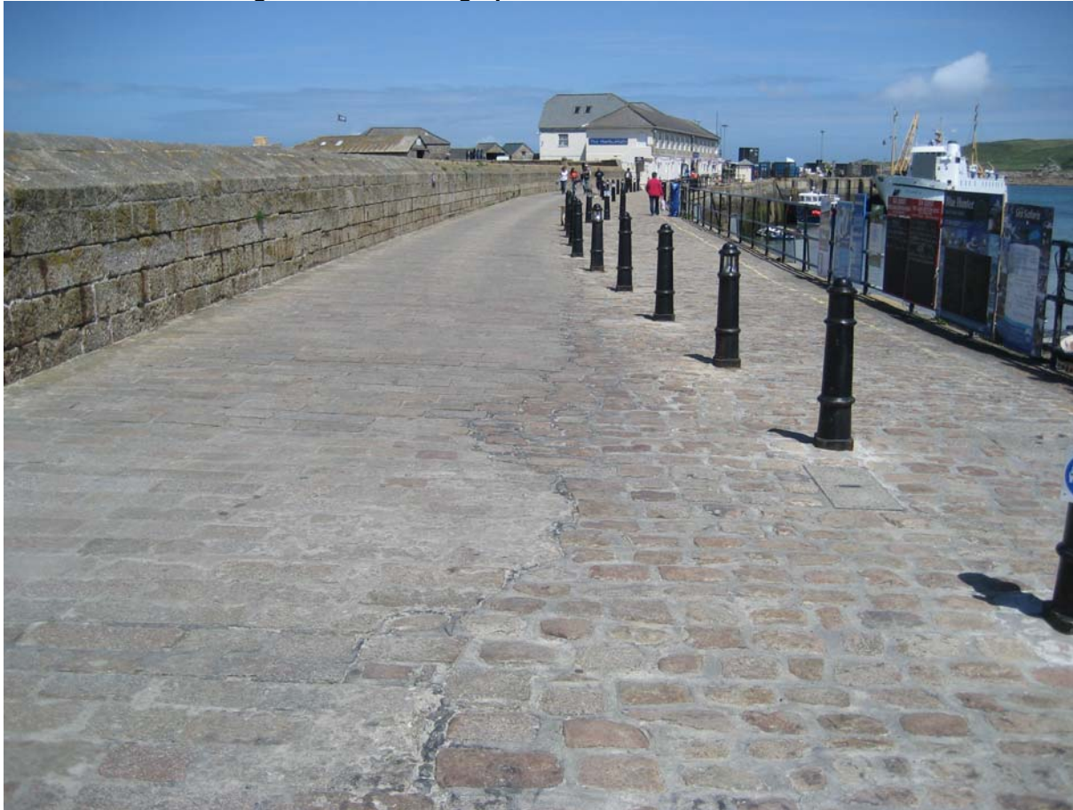
Existing view of quay surfacing looking north. Granite flagstones are to the left (west), granite setts are to the right (east), separated by a line of pedestrian bollards.
