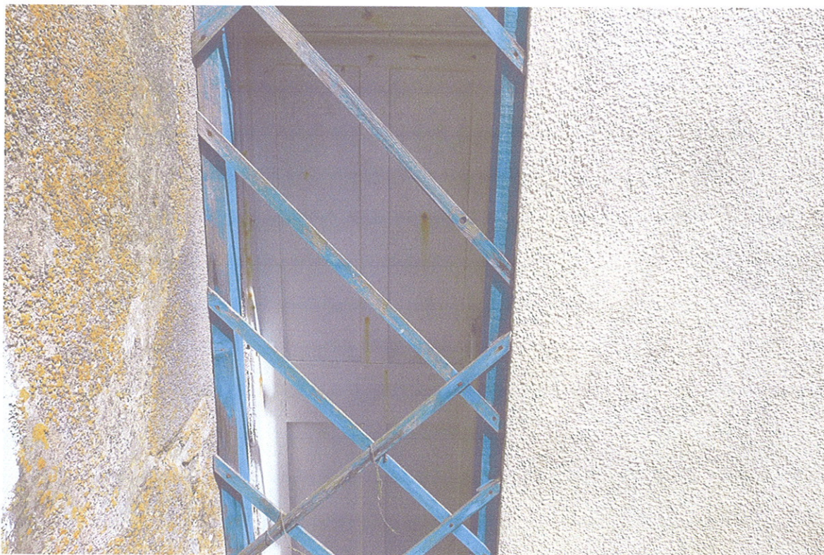
REAR ENCLOSED DISUSED DOOR.
