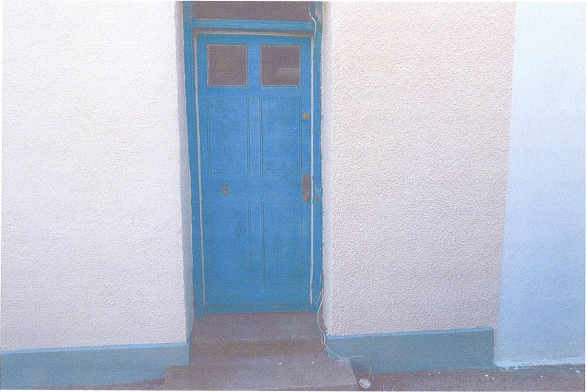
FRONT DOOR ON TO BUZZA STREET
