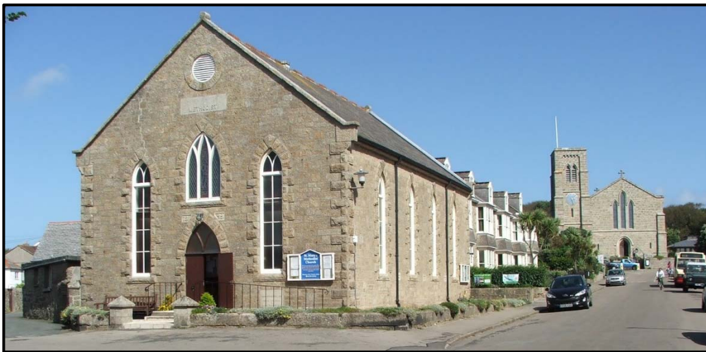
Image 7 - St Mary's Methodist Church (Church Street)
