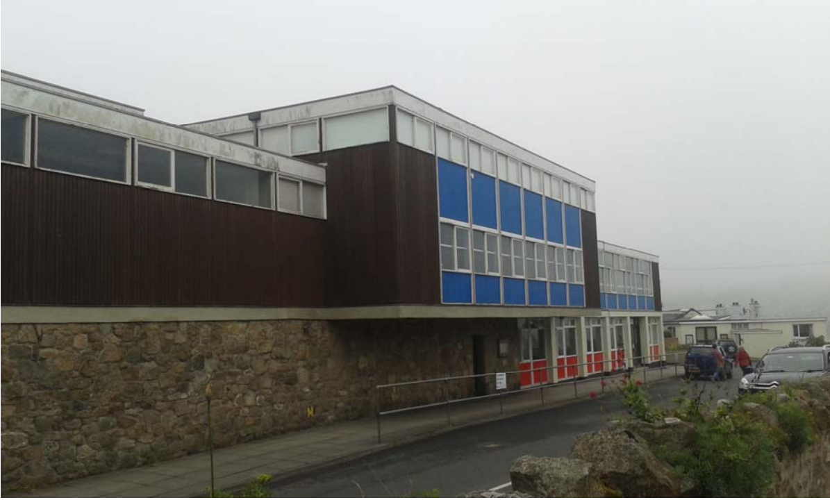
View of the western block
