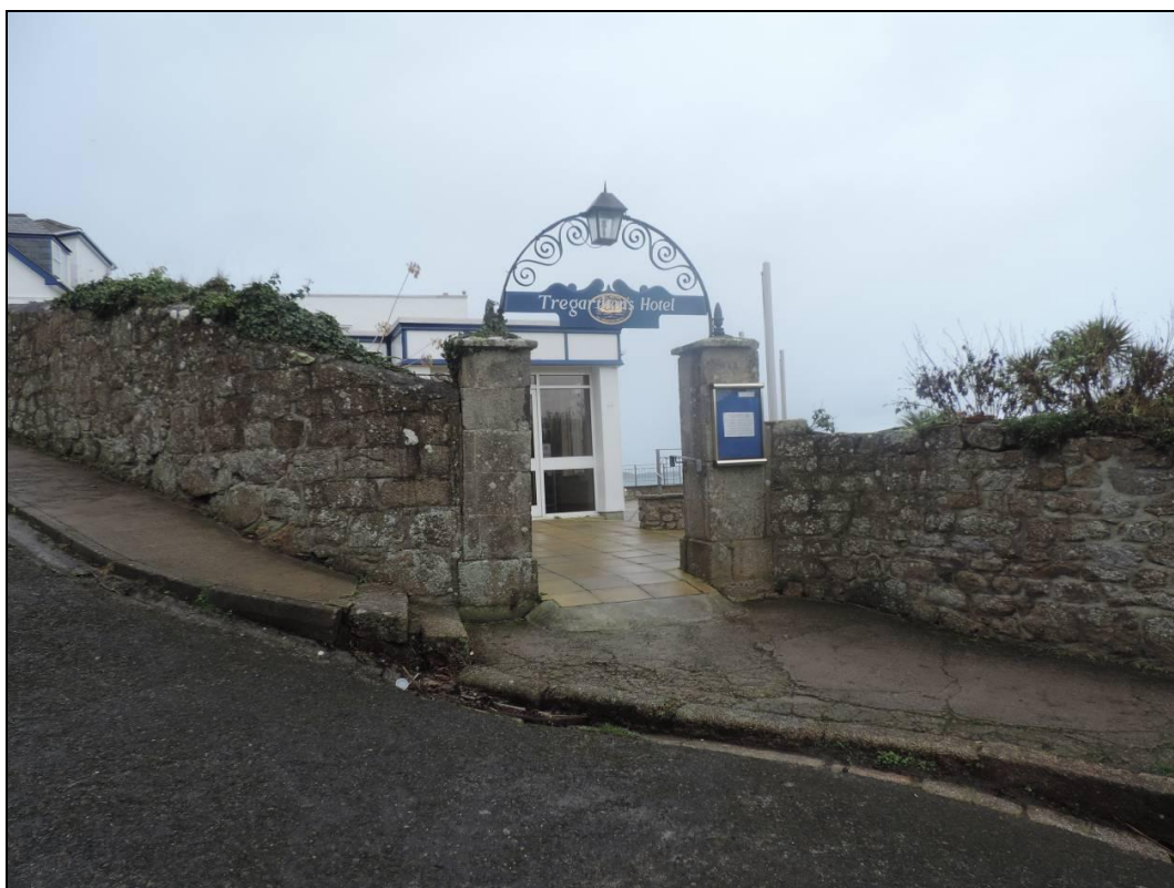
5. View of Garrison Hill pedestrian entrance
