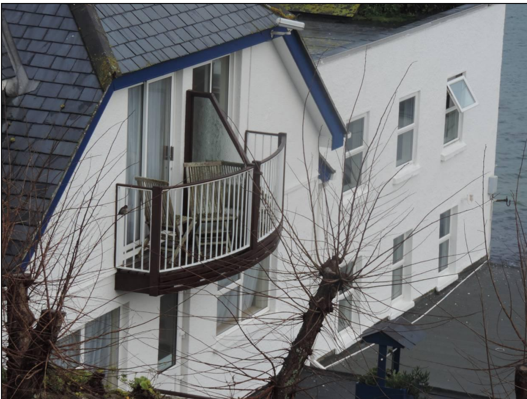
4. View of southeast side upper level from Garrison Hill
