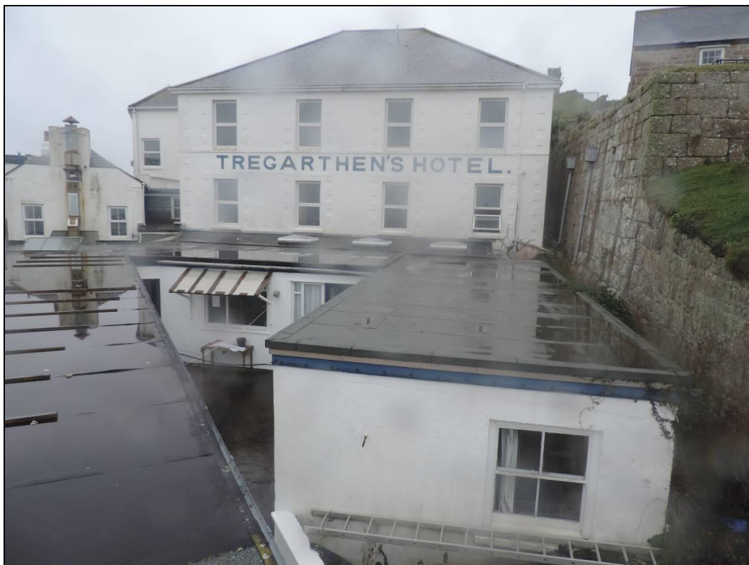
9. View of north elevation over low level staff accommodation.
