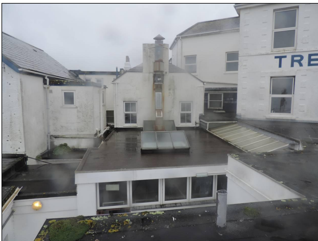
8. View of multiple roof structures to building core.
