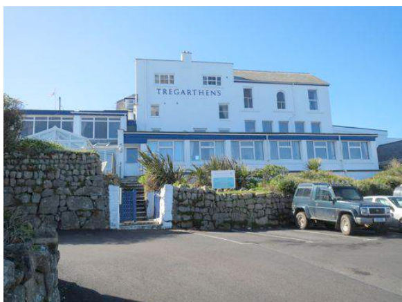
Photograph 1. Front (north) elevation of Tregarthens Hotel
