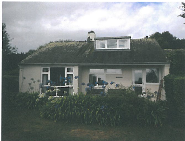
Existing view looking from the east
