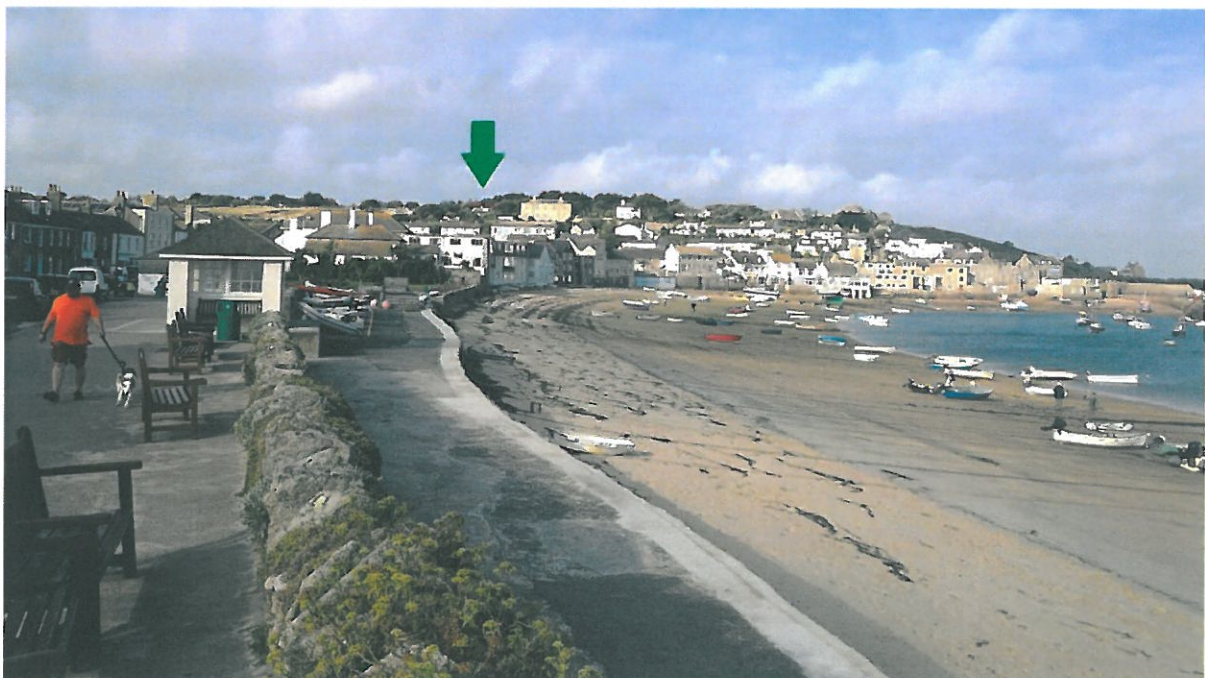
Photo 2 [Taken from eastern end of the Strand]
