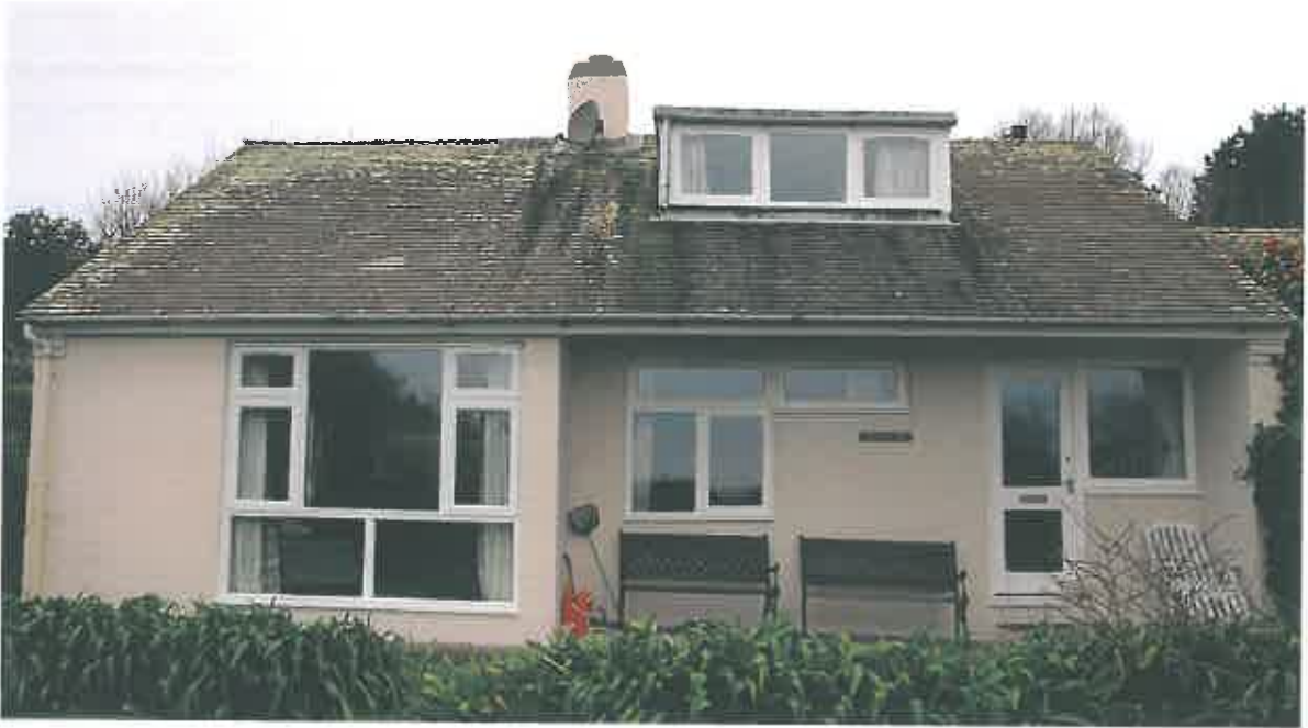
Fig 12 East facing elevation of Tamarisk.
