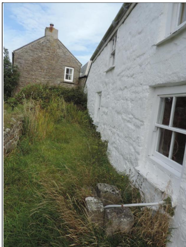
2. View along north elevation looking east.
