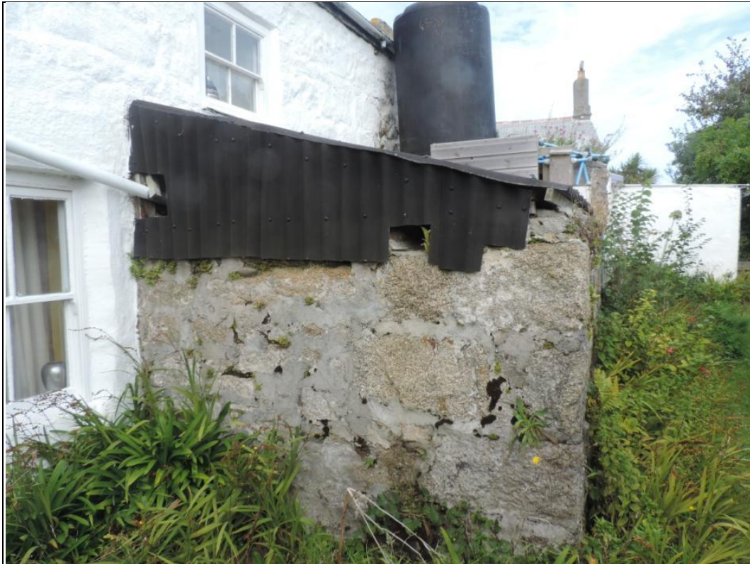
7. View of tank store.
