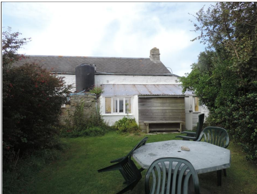
5. View of south elevation.
