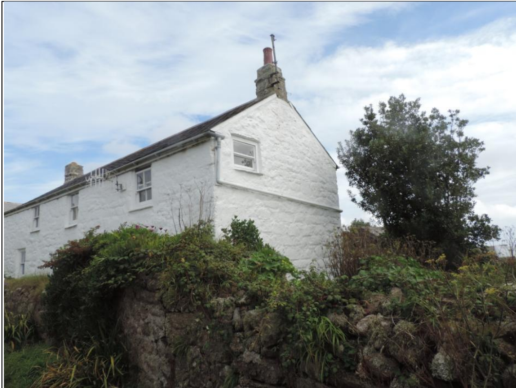
3. View of west end.
