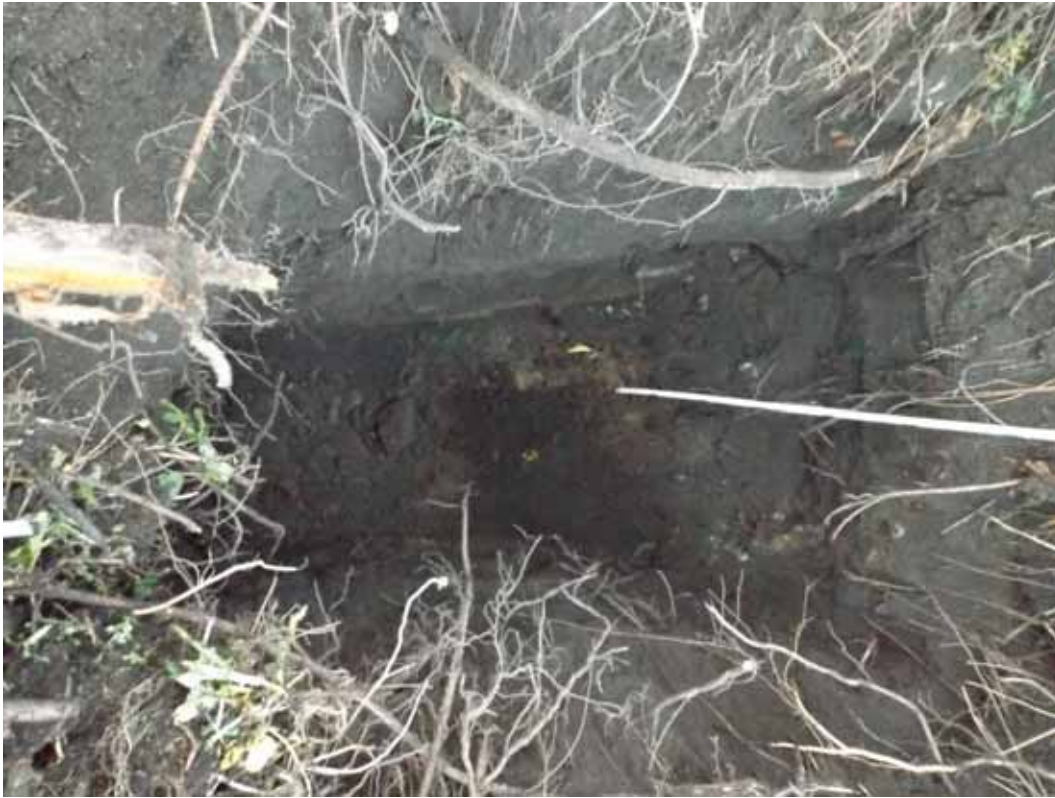
Plate 11: Geotechnical test-pit at west end of garden area. There is a single homogenous layer of dark garden soil lying above the ram, the weathered top of the underlying granite.
