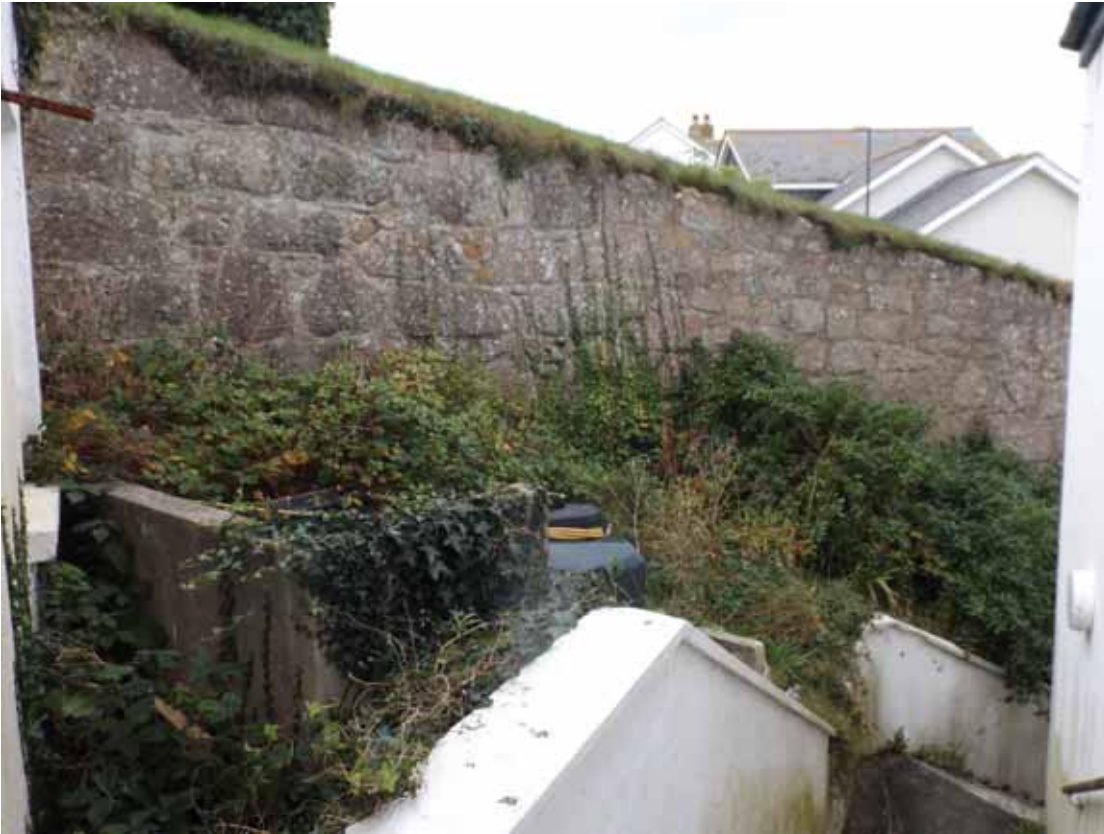
Plate 9: Detail of the curtain wall masonry.
