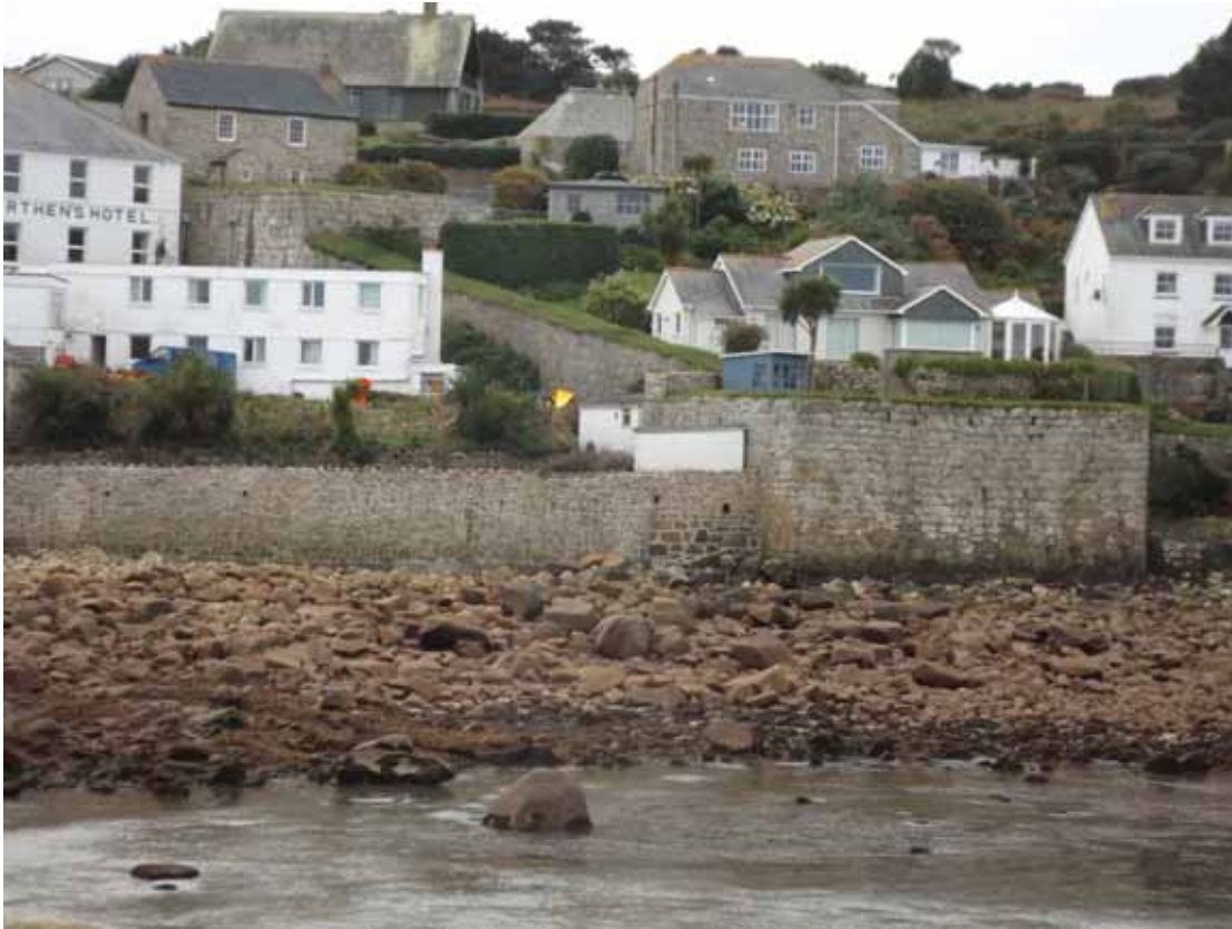
Plate 5: Detail of the Gunners Well Battery, the sea wall, and the curtain wall (turf-capped) rising to the gatehouse.
