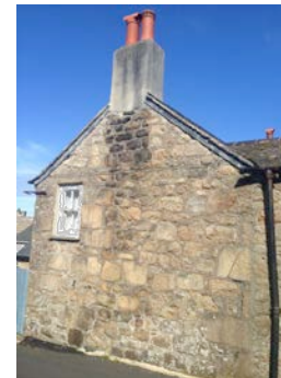
Local stone gable ends
