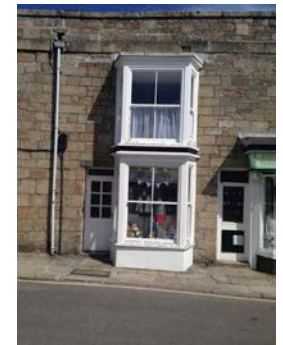
Two storey bay windows
