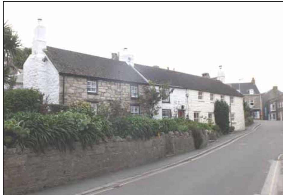
Plate 21: Crows Nest, The Cabin and The Forecastle, viewed looking northwest
