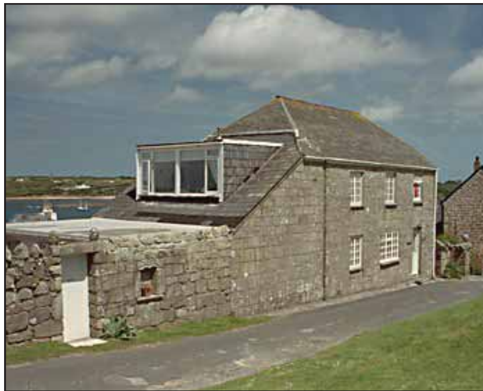
Plate 10: Garrison Cottage, looking southeast (source: Images of England)
