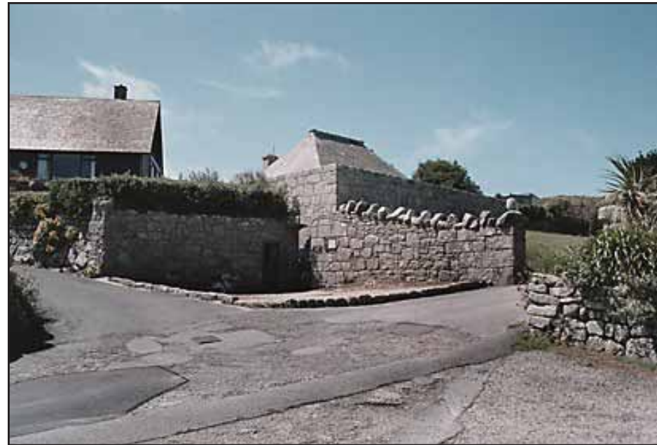
Plate 7: The Rocket House, Powder Magazine and Blast Walls
