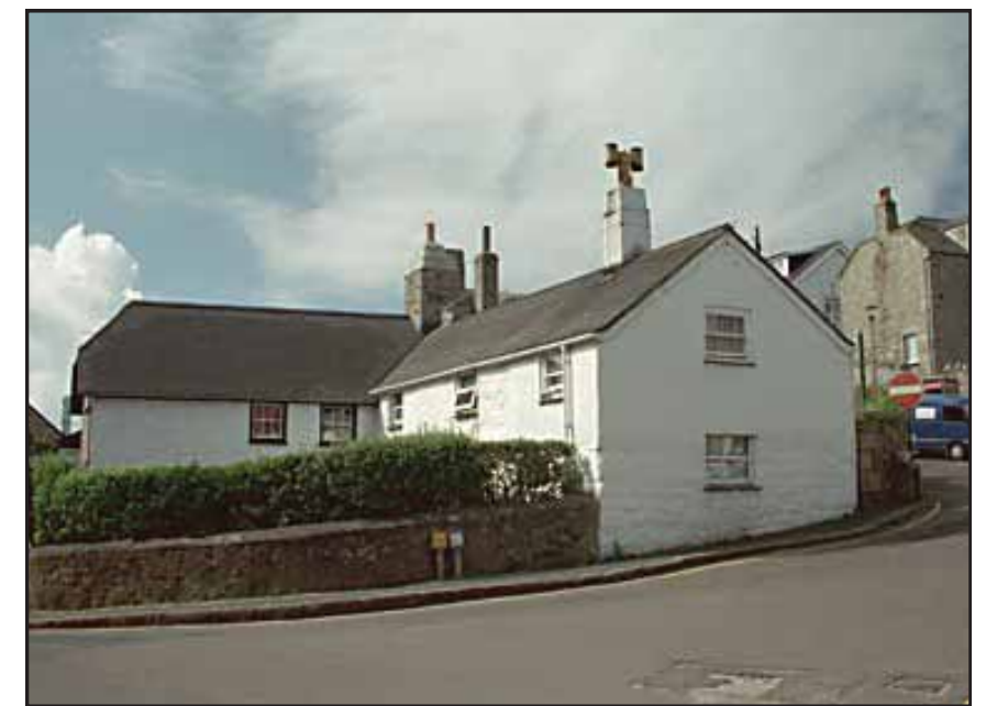
Figure 20: Dolphin Cottage, viewed from Hugh Street, looking south (source: Images of England)
