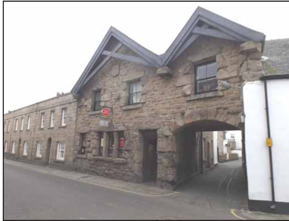
Plate 26: The Post Office, Hugh Street, viewed looking southeast
