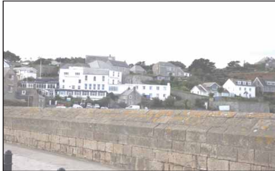
Plate 2: Tregarthen's Hotel viewed on the Pier from the northeast
