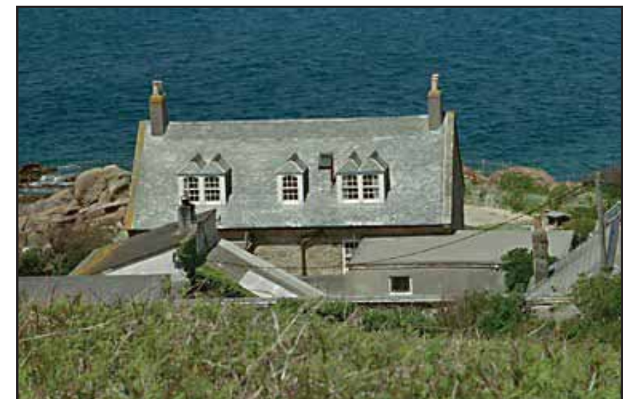
Plate 12: Newman House, looking north (source: Images of England)
