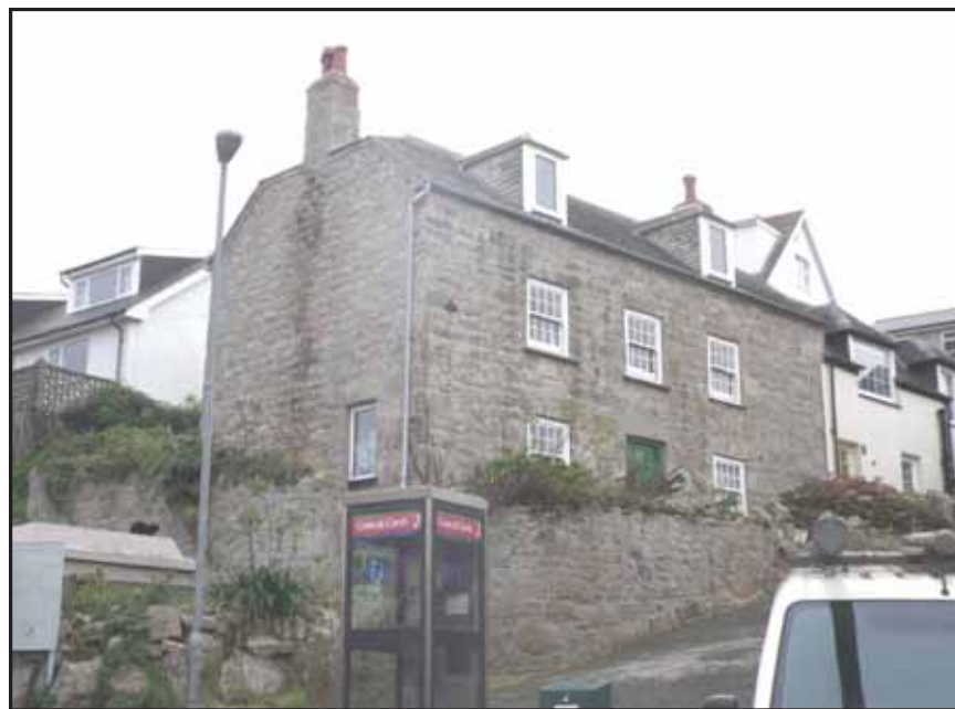
Plate 15: No.3 Garrison Hill looking southwest
