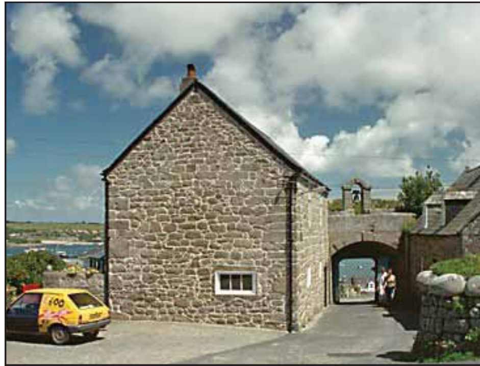
Plate 9: The Guard House, looking southeast (source: Images of England)
