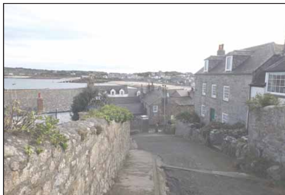
Plate 16: View down Garrison Hill towards Hugh Town, Dolphin Cottage rear façade to centre of image
