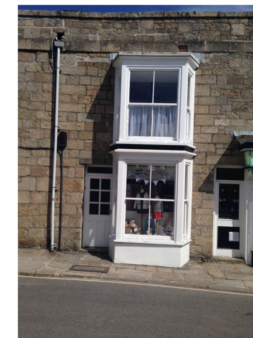
Two storey bay windows
