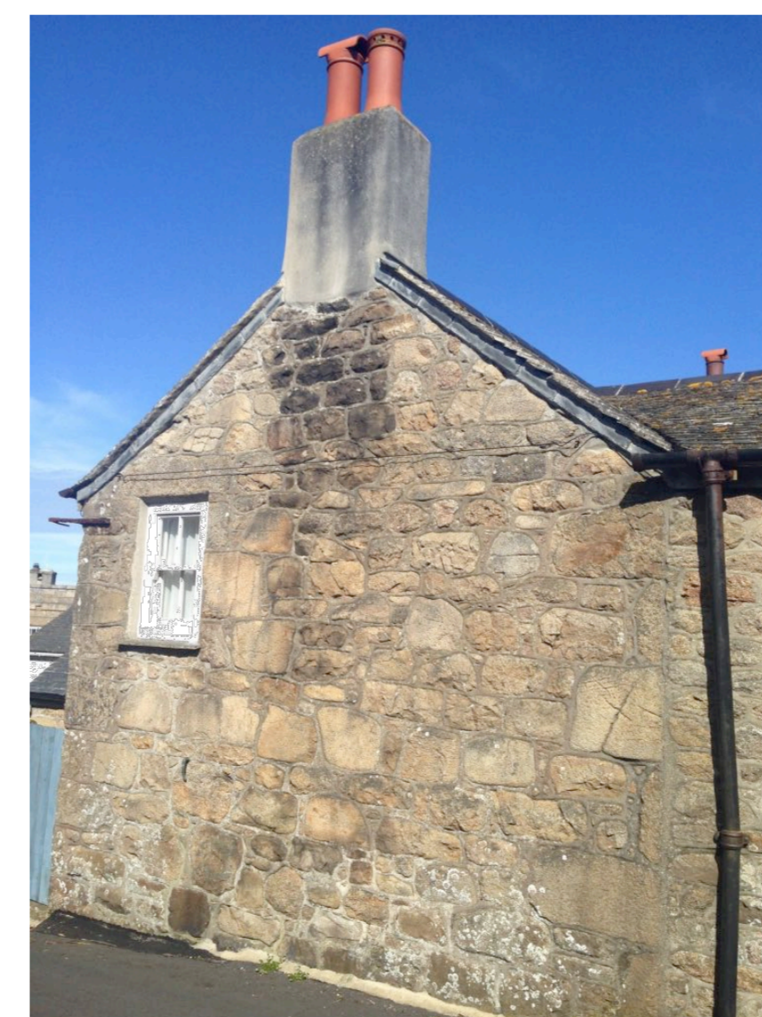
Local stone gable ends
