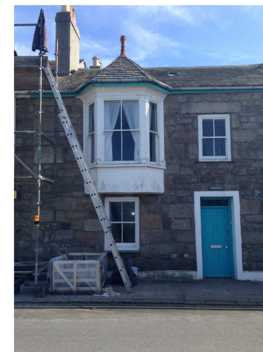
Bay windows breaking the roof line
