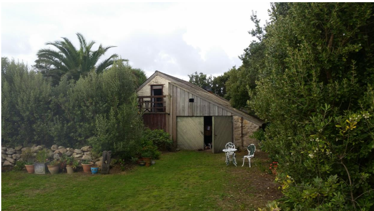
Fig. 1: East elevation of The Boathouse, Green Bay, Bryher, Isles of Scilly
