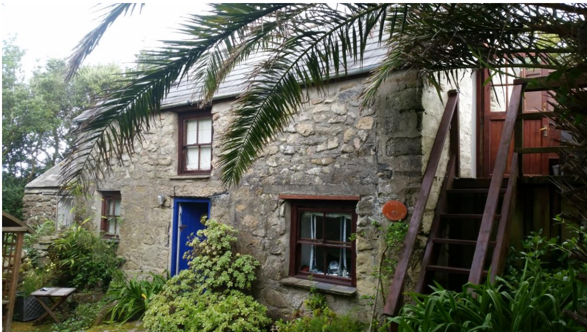
Fig. 2: South elevation of the cottage, The Boathouse, Green Bay, Bryher
