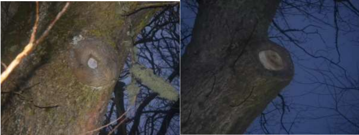
Fig 1.1 Two examples of correctly sited pruning cuts on Elms, showing good callousing and healing following the cut and no signs of rot or fungus
