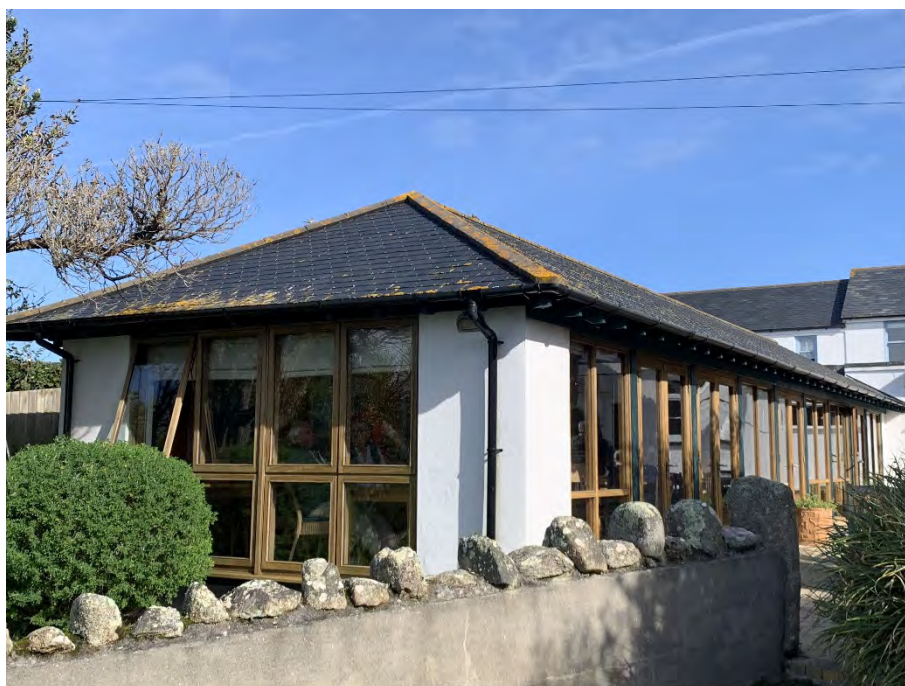
Figure 1: View of south west and south east elevations of dining room.
