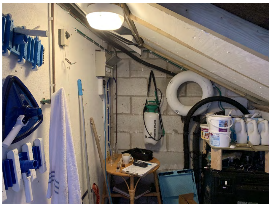
Figure 4: View of interior of chemical store.
