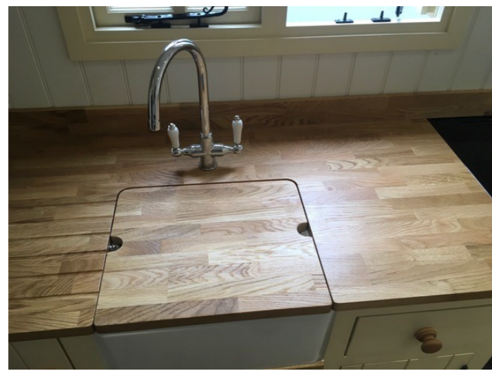
Kitchen (illustrative) Hardwood worktop and butler sink unit with tongue-and-groove wood-clad walls and window to allow natural light as well as ventilation during cooking and food preparation
