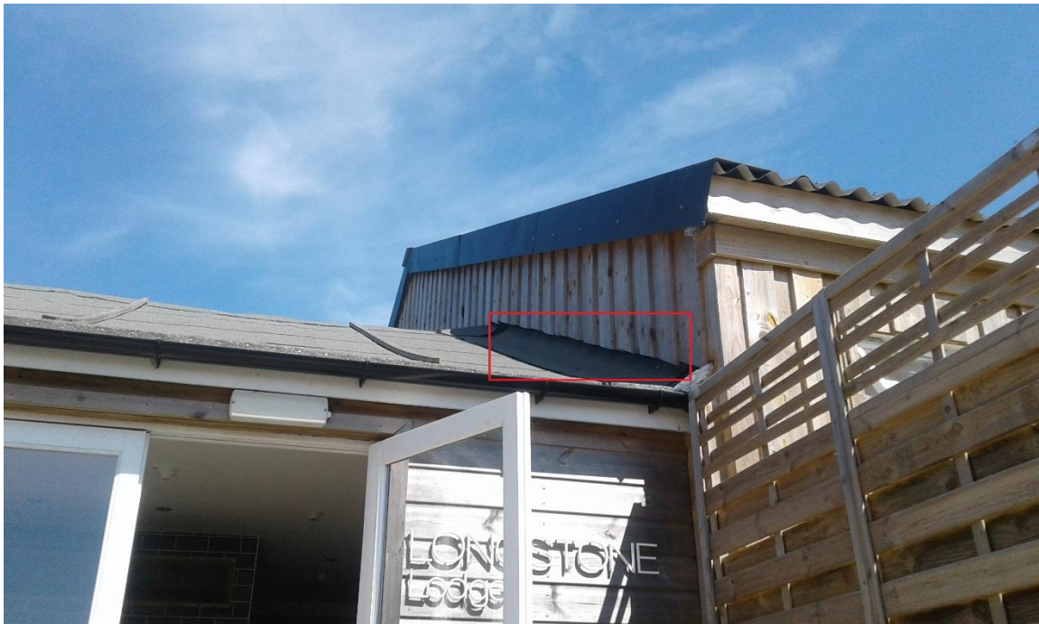
Photo 9. The hit and miss timber arrangement creates voids with access below.
