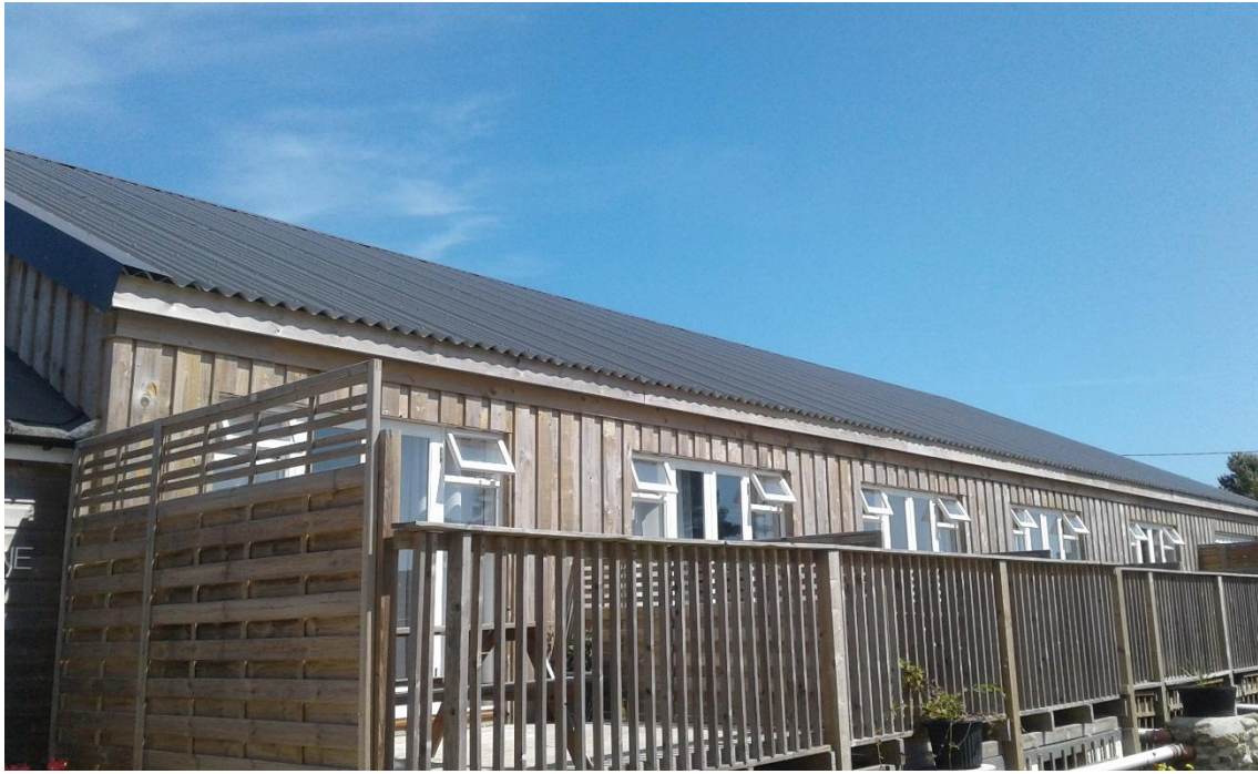
Photo 1. Longstone Lodge (south aspect)
