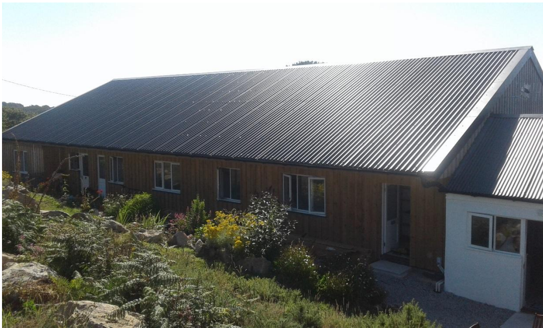
Photo 2. Longstone Lodge (north aspect).
