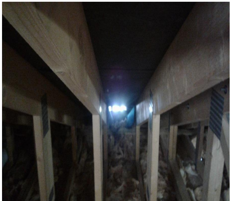
Photo 12. Natural light entering loft space.
