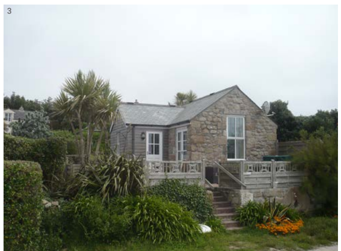
1 Stone Annexe to the right of the house, viewed from the garden 2 Timber workshop at the foot of the garden 3 The Moorings, accessed from the beach path
