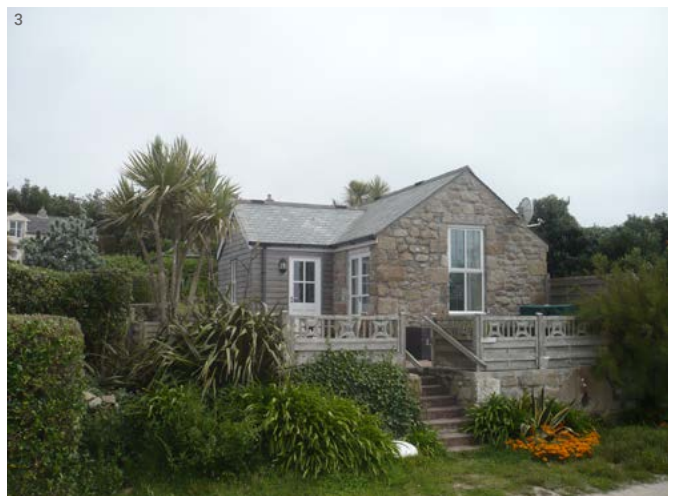
1 Stone Annexe to the right of the house, viewed from the garden 2 Timber workshop at the foot of the garden 3 The Moorings, accessed from the beach path
