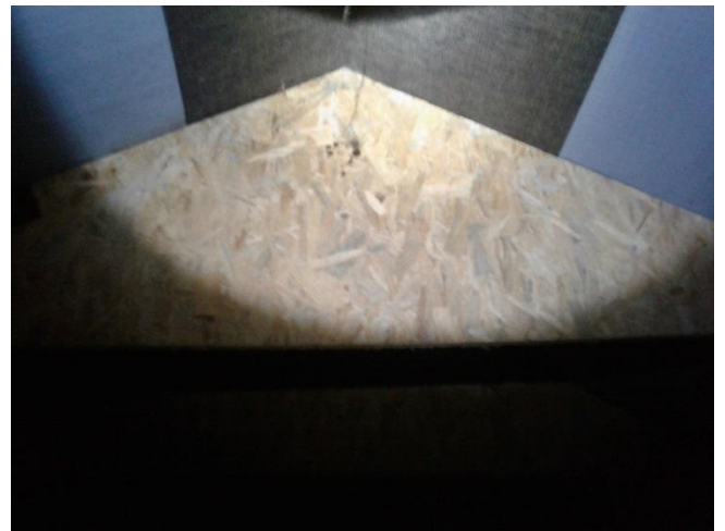
Photo 24 – Chipboard above collar beam.
