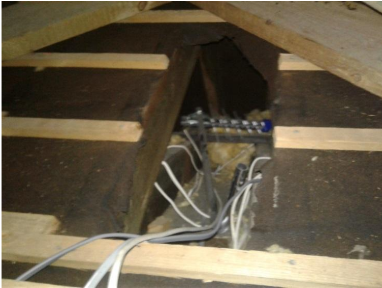
Photo 22 – End of the loft partially partitioned off.
