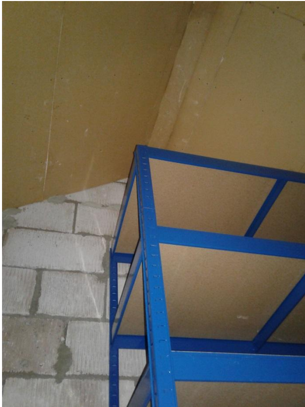
Photo 18 – Loft space in south-east end of main house.
