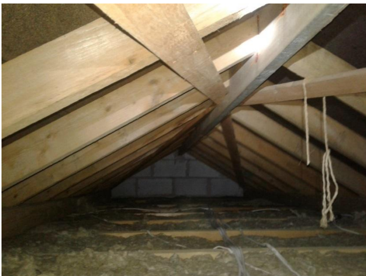
Photo 19 – Loft of gabled extension.
