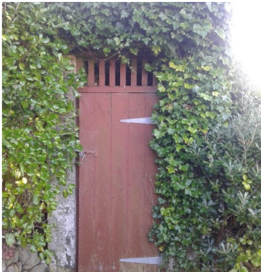
Photo 4 - Small standalone shed (north-east aspect).
