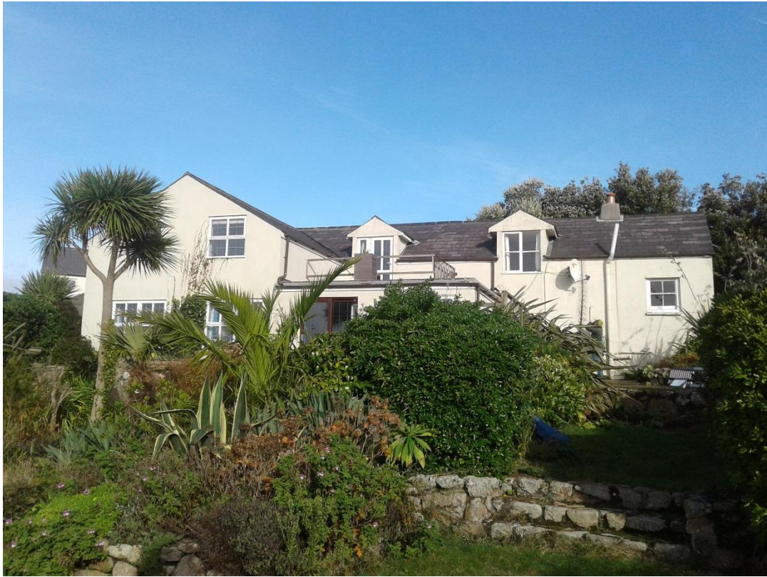
Photo 1 - The main house (south-west aspect).
