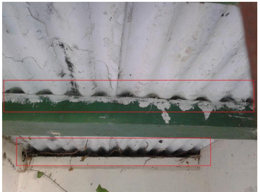
Photo 30 - Inside the small standalone shed.
