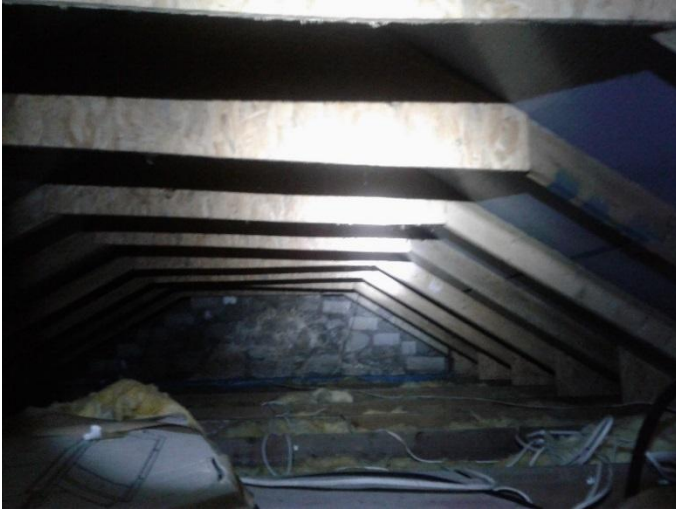
Photo 23 – Cottage loft space.
