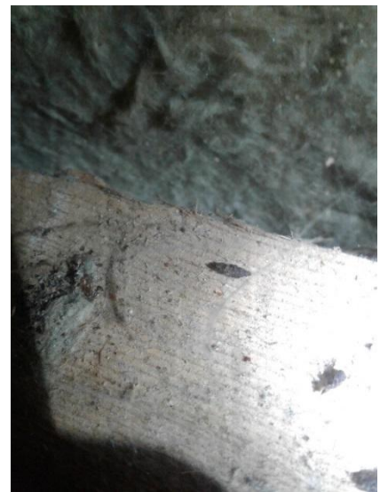
Photo 20 – Dropping on beam.
