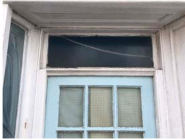
Over Door Glazing and Door Frame (From Street)
