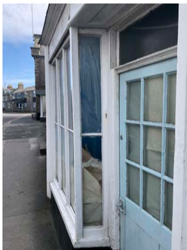
Window and Door Frame mouldings, Corner of Window Frame shown is a later addition to reinforce window structure (As shown in Carpenters diagram)
