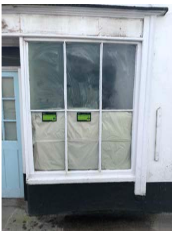
Right Front Window (Seen from Street)
