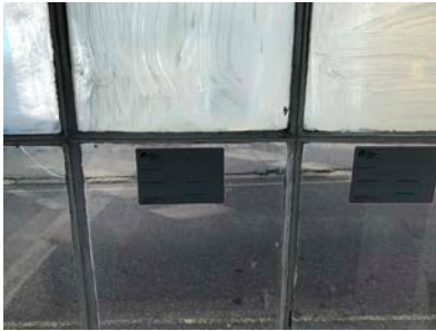
Window Moulding (Inside View) Showing internal Putty to Glazing
