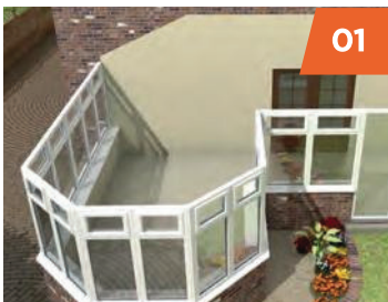
01 The vital first step is to remove the entire existing roof.
