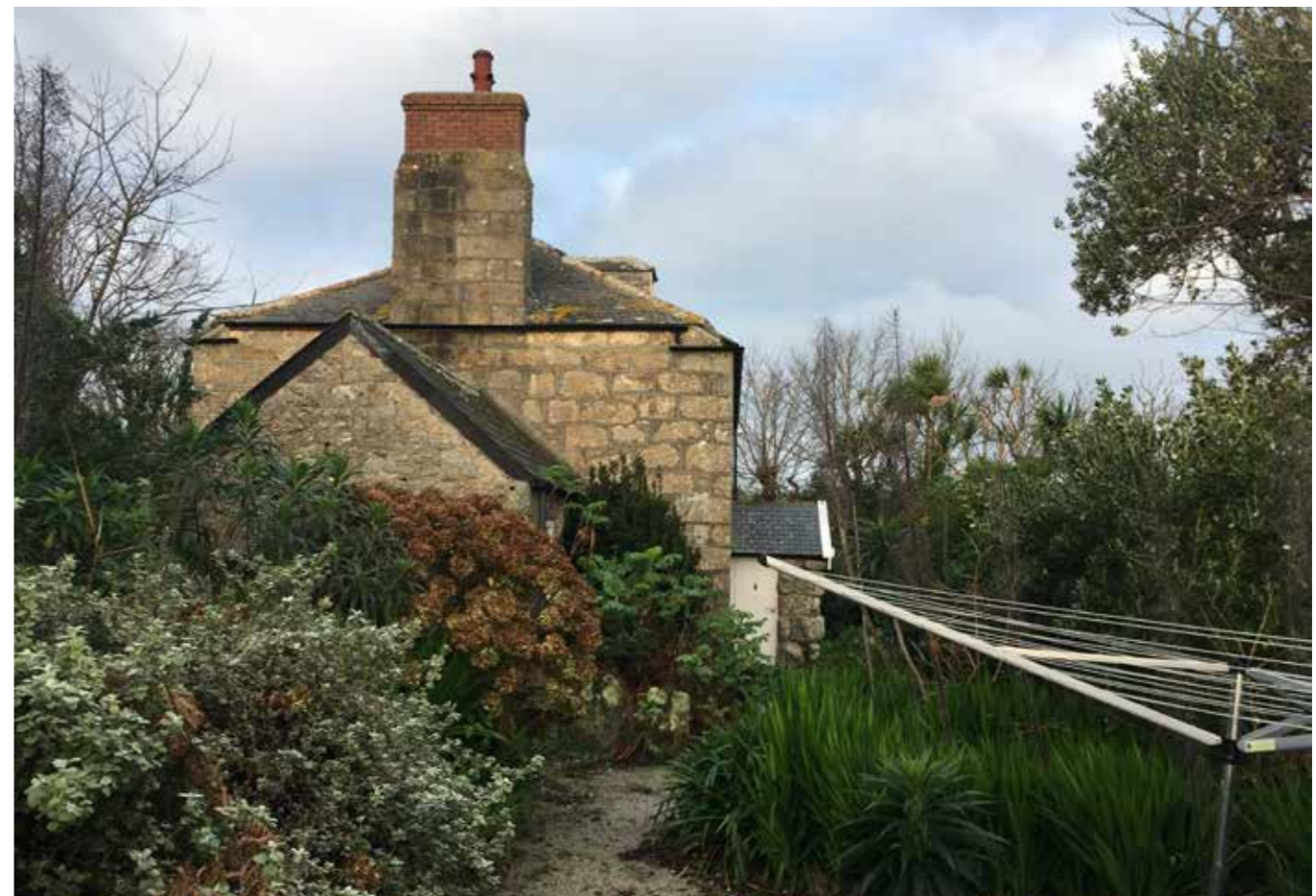
Figure 9 - South east elevation of Dolphin House (LHL)
