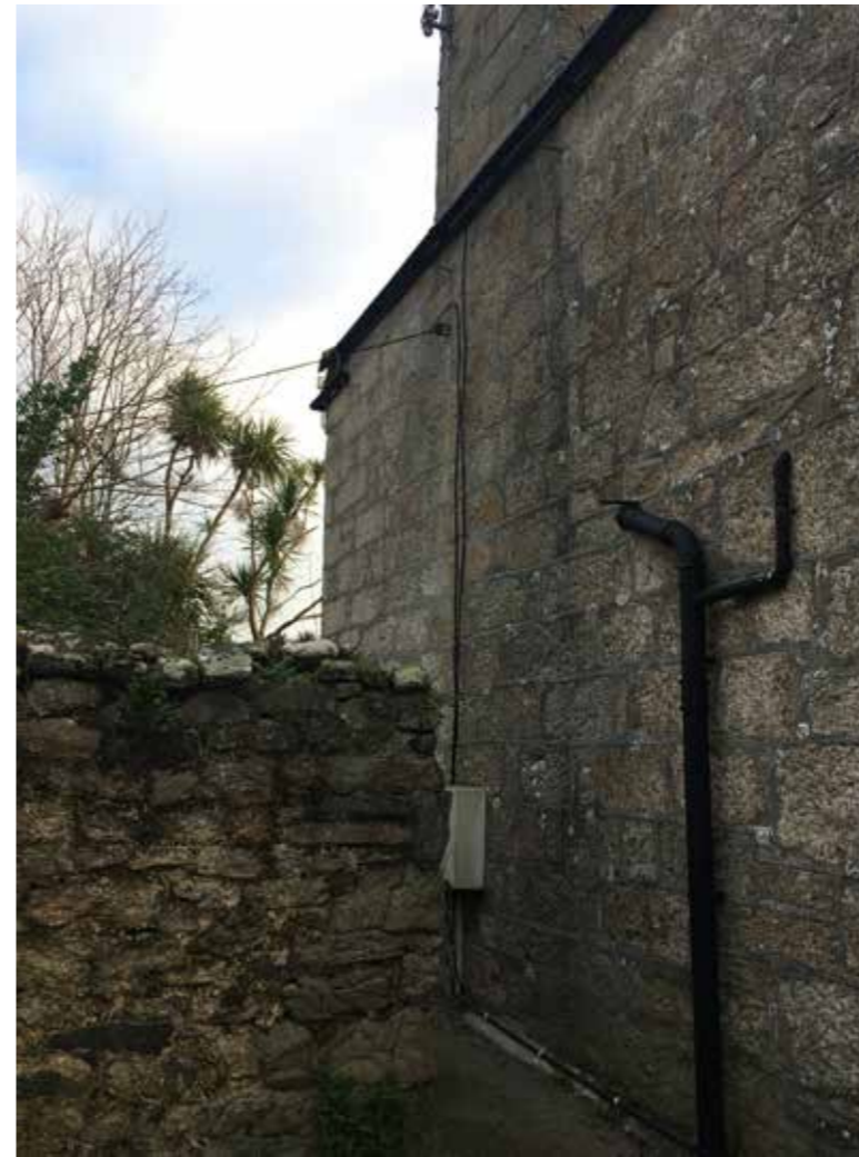
Figure 8 - North west elevation of Dolphin House (LHL)
