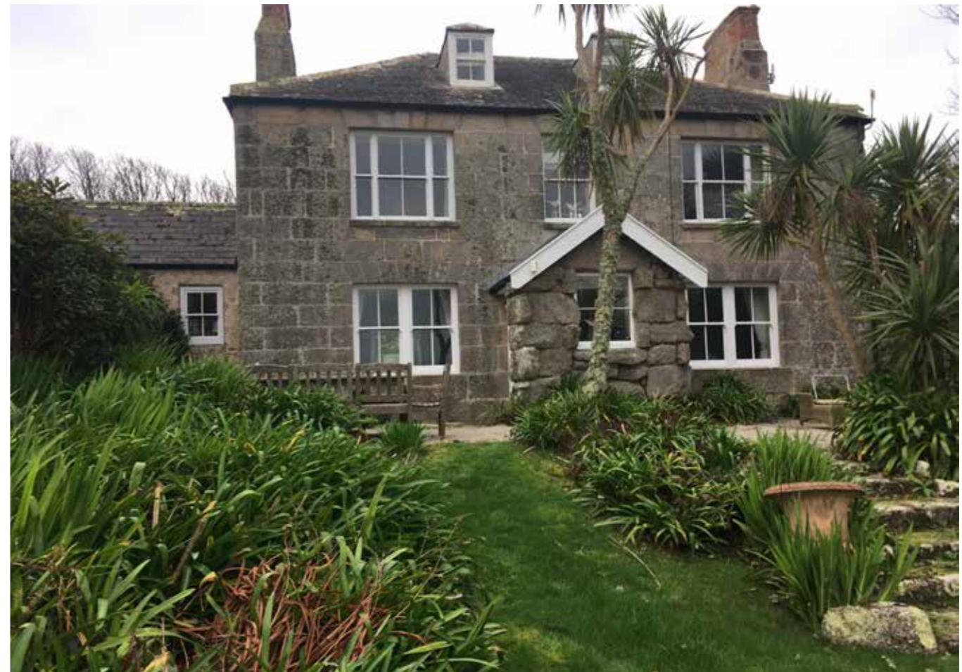
Figure 6 - Front elevation of Dolphin House (LHL)
