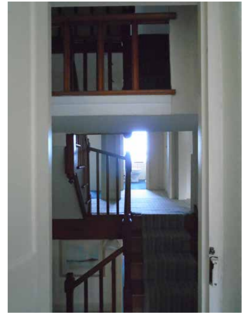
Figure 16c - View to first floor landing with half landing to the attic above
