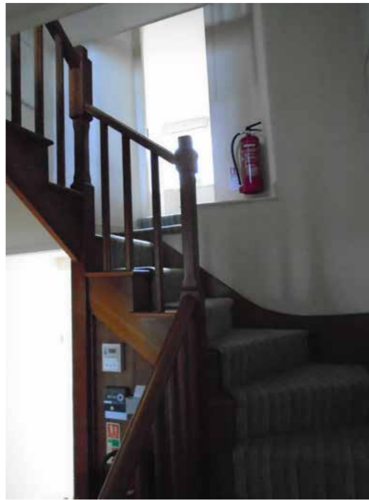
Figure 16b - Staircase ground to half landing and access to rear extension
