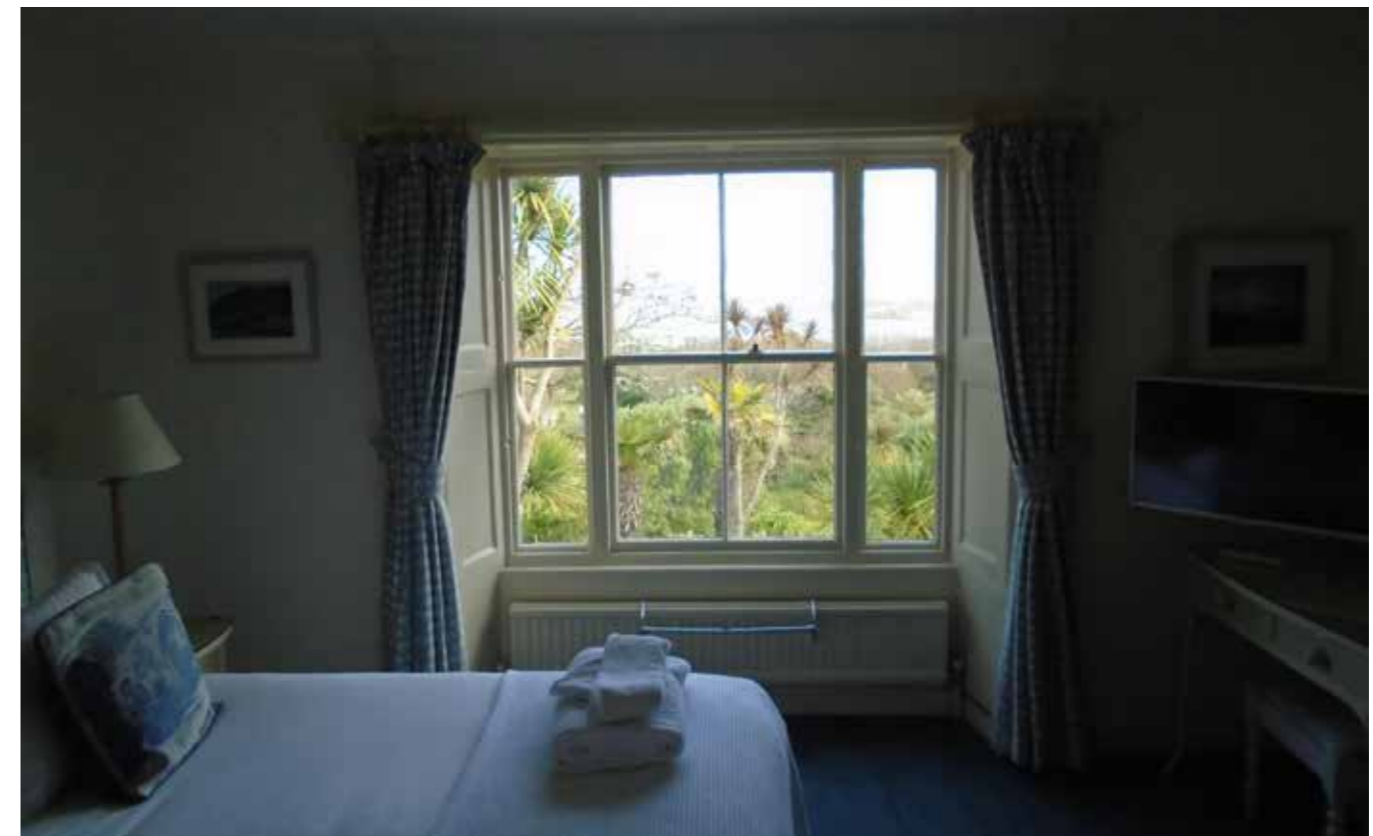
Figure 15 - Original window joinery in bedroom 2 (Tresco Estate)
