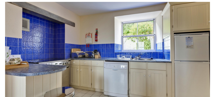
Kitchen, Note; uPVC window; C20th fitting and finishes; alterations to chimney breast
