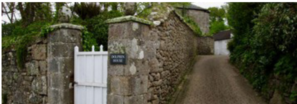
Wall and gate separating front and back of house approaches
