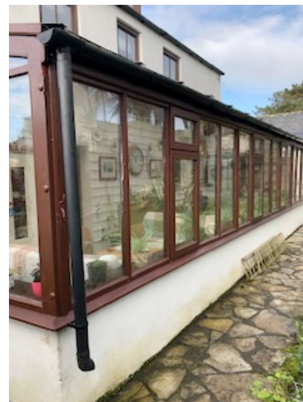
Images showing the existing conservatories
