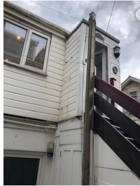
existing porch and rear cladding in UPVC
