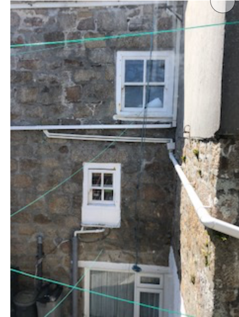
mixture of timber and UPVC windows to rear of The Anchorage
