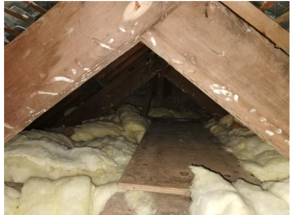
Photo 6. Showing roof void over the main part of the cottage
