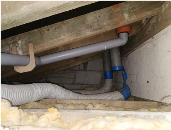
Photo 5. Showing roof void over the lean-to
