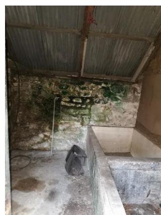
Photo 8. Showing the western room in the outbuilding
