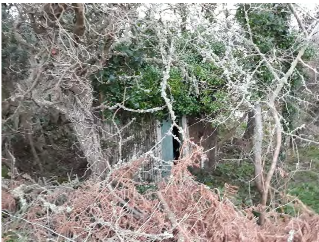
Photograph 14: Pump house, adjacent SW corner of site (to WSW).
