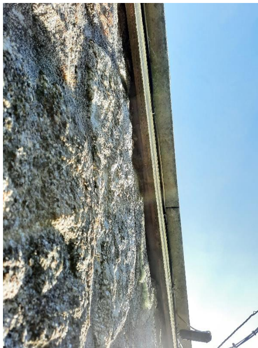
Figure 5: View of gaps beneath the timber fascia board.
