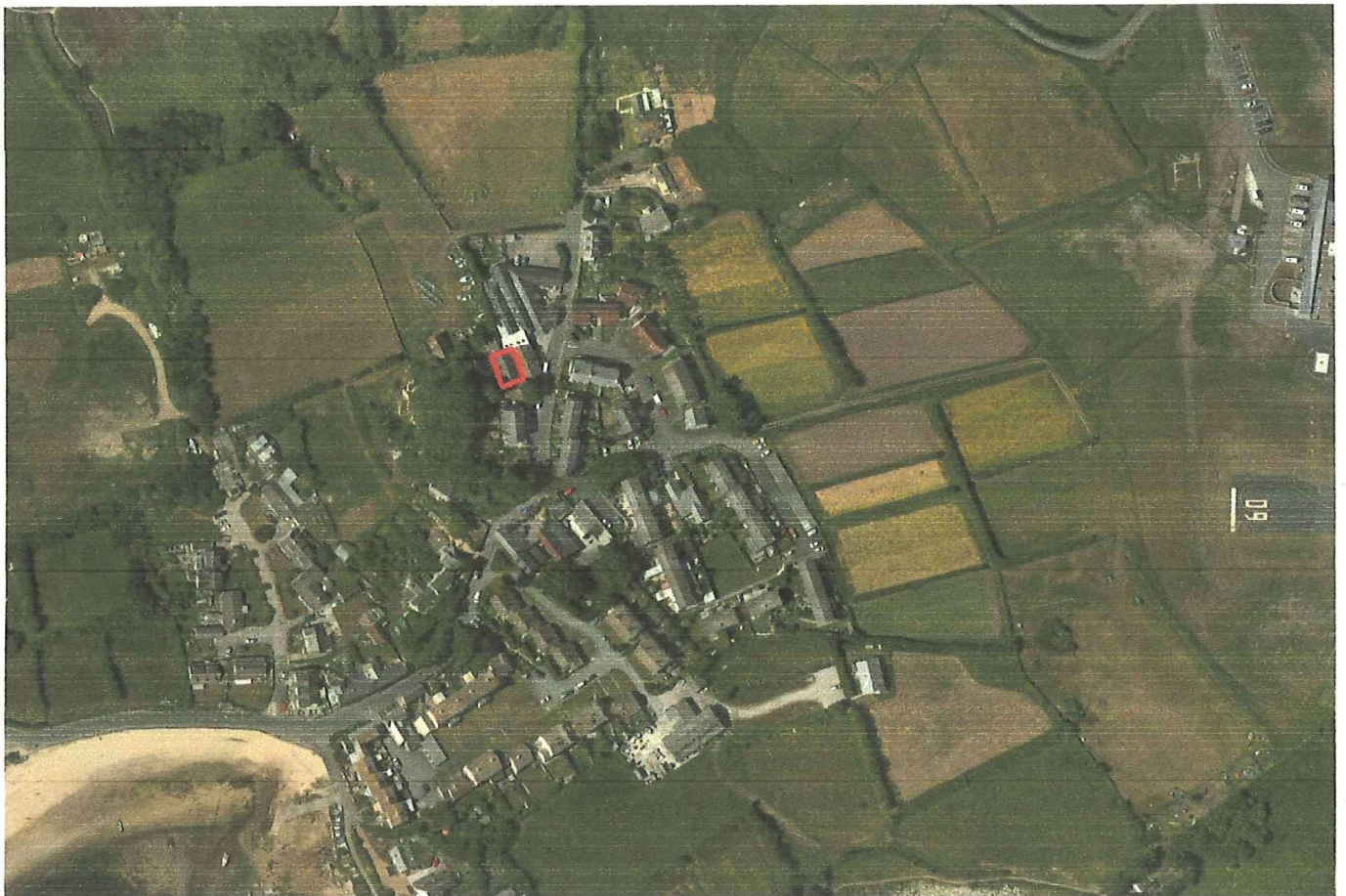
Figure 1. Castle Farm Workshop general location
