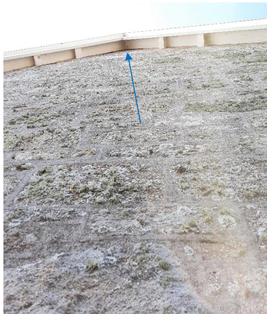
Figure 6: View of gaps beneath the timber soffits on the northern gable end at The Moorings (shown by the blue arrow).
