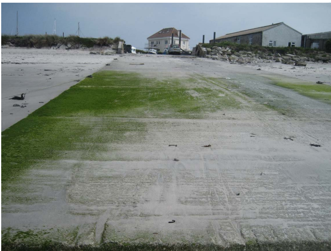
Figure 4-3: Slipway constructed at Porthloo in 2014
