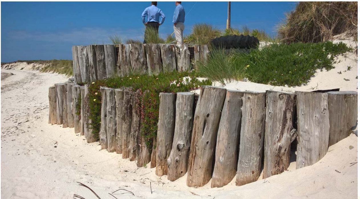
Figure 4-26: Localised defence works on South Dunes
