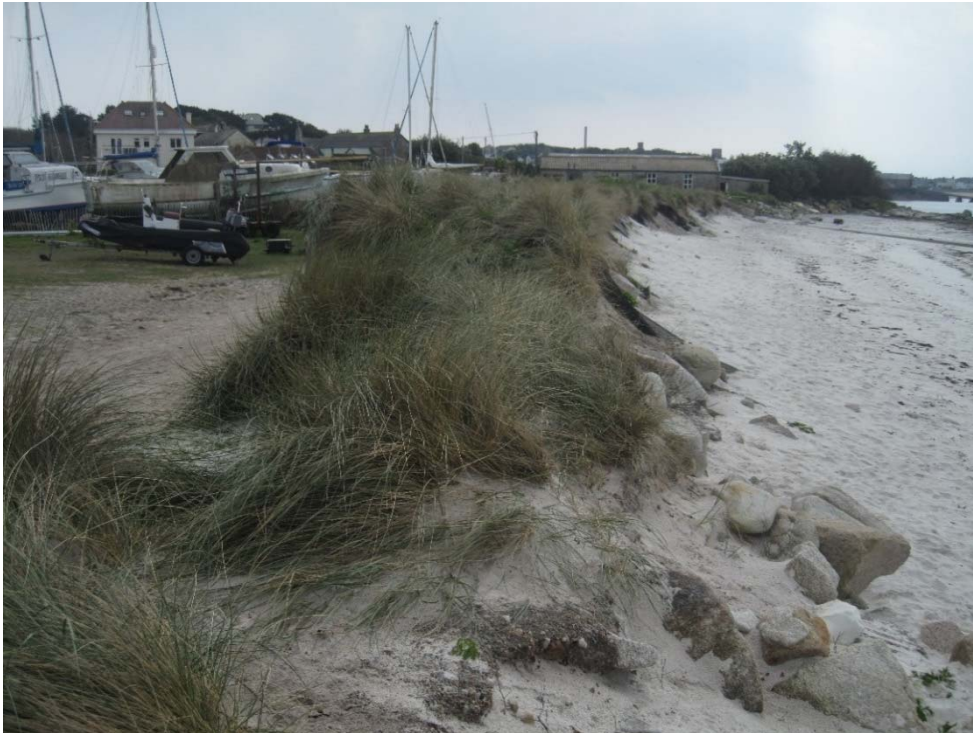
Figure 4-16: Rubble partially covered in sand in northern part of bay
