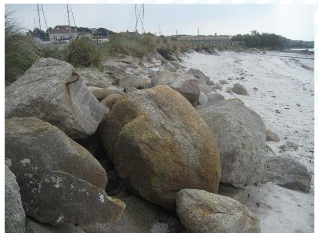
Plate 2: View of Porthloo beach looking south, with rock rubble defence in the foreground and exposed dune stabilisation works, concrete slipway and boat yard in the background
