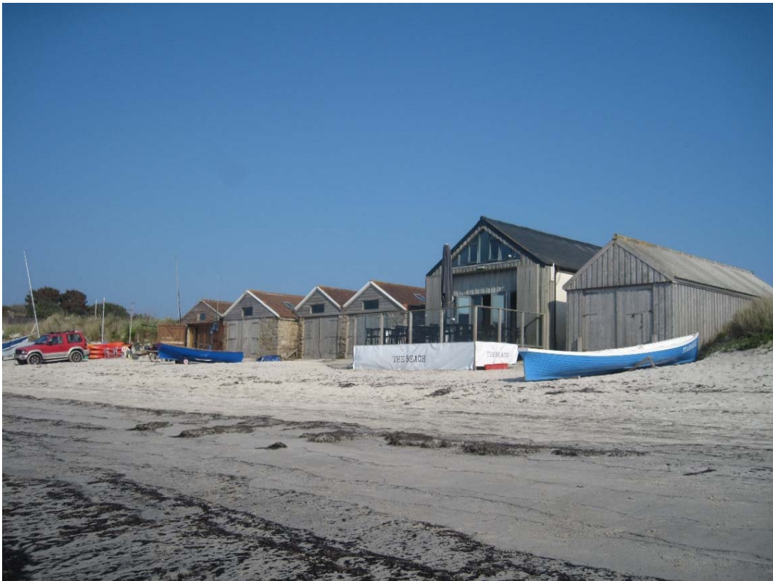
Figure 4-5: Buildings encroaching onto beach at Porth Mellon
