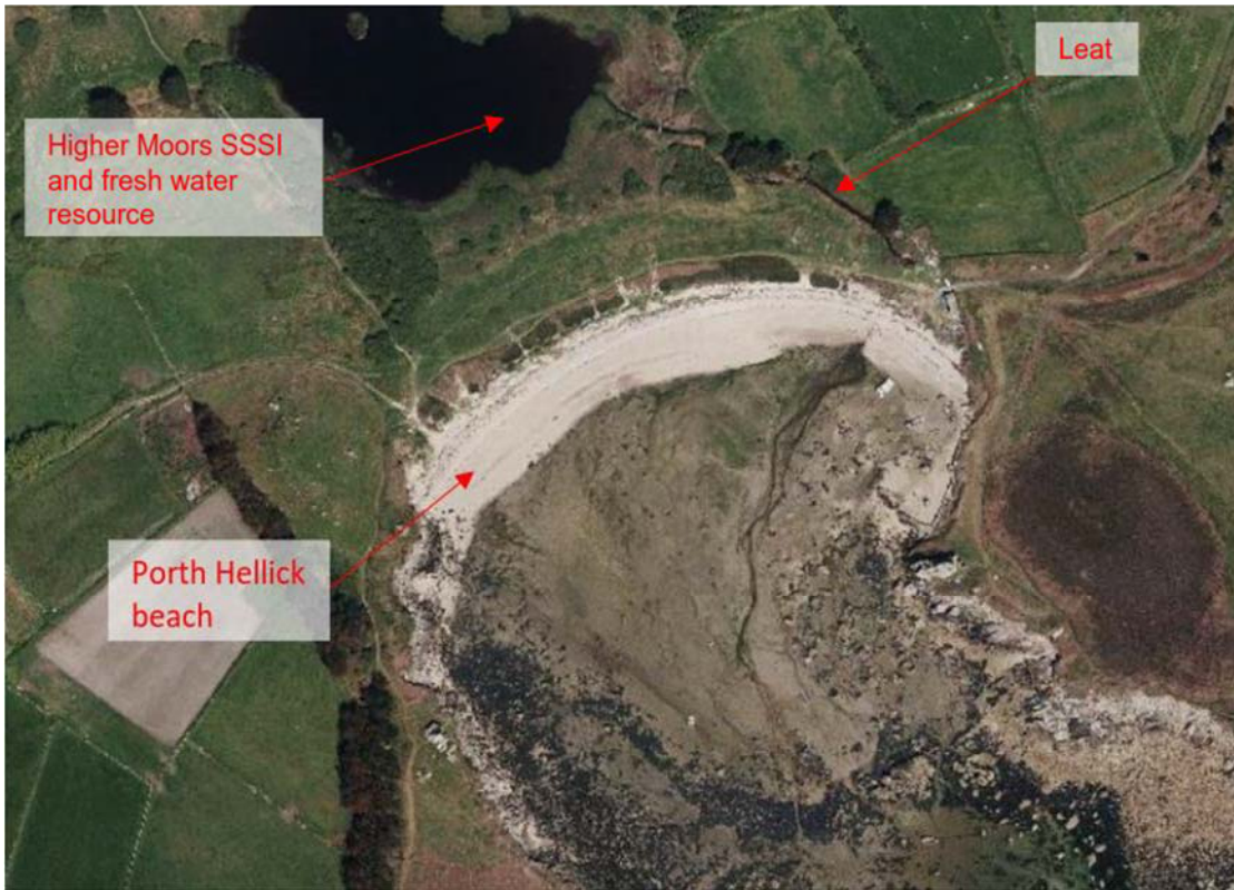
Figure 4-8: Aerial imagery showing Porth Hellick Beach and Higher Moors SSSI
