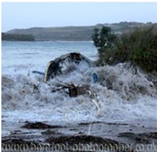
Figure 4-31: Breaching of the slipway during 2014 storms 22
