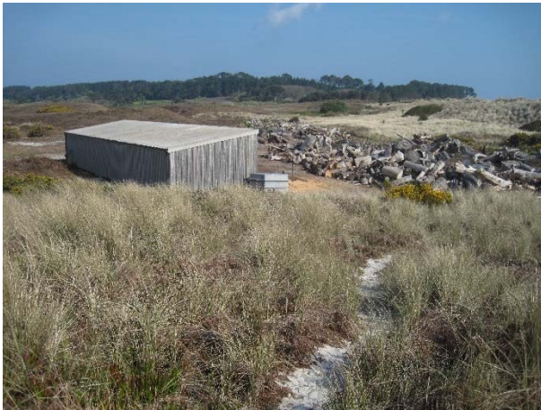
Plate 15: Timber wood store and building located immediately landward of the dunes, next to the telecommunications junction box
