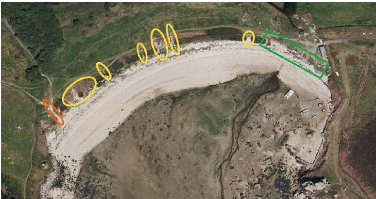
Figure 4-22: Vulnerable zones of weakness on Porth Hellick beach crest
