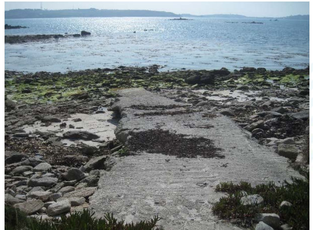
Plate 16: Existing concrete access ramp at the western end of South Dunes beach
