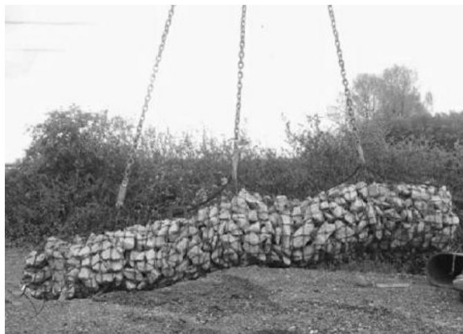
Picture 1 - showing lifting points
