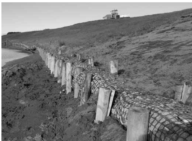
Picture 2 - showing staking technique
