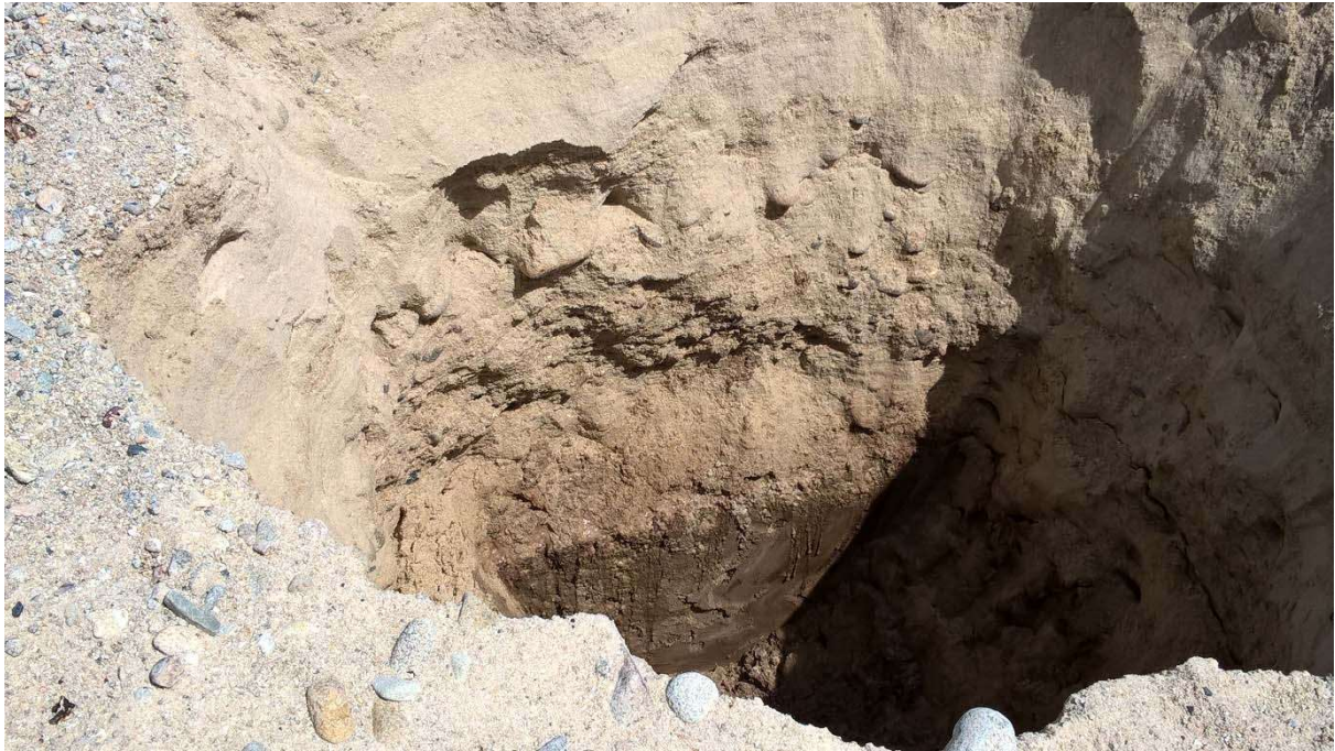
Fig 6 – Pit 3, South Beach – note water seepage at boundary between sand and claystone
