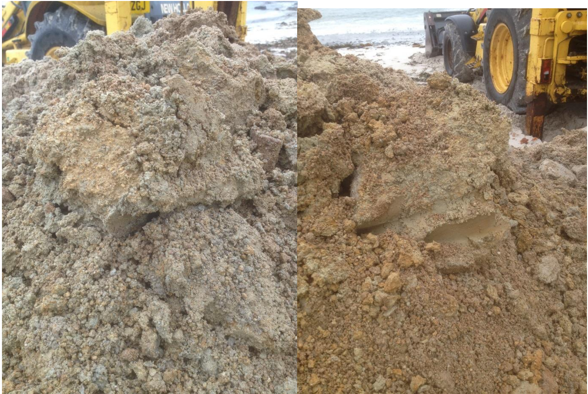
Fig 3 and 4 - Pit 1 mix of lumps of clay and ram from spoil heap
