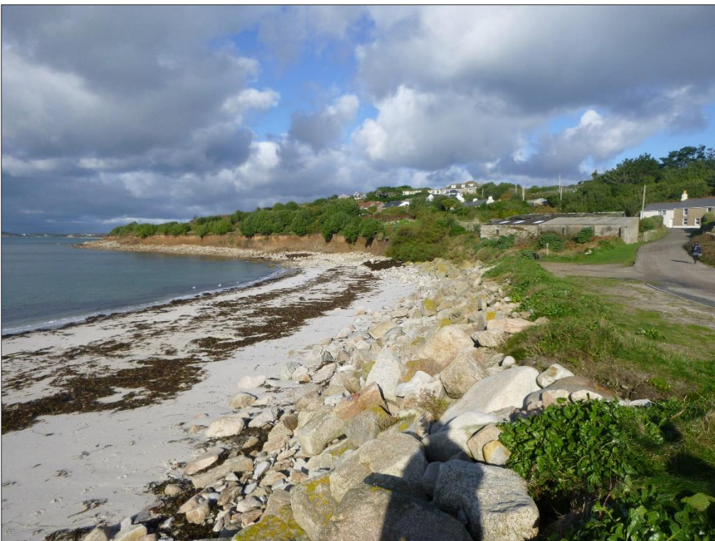
Figure 3: Looking toward the northern end of the beach. Note existing granite rock forming an ad-hoc revetment and Porthloo lane behind the beach.
