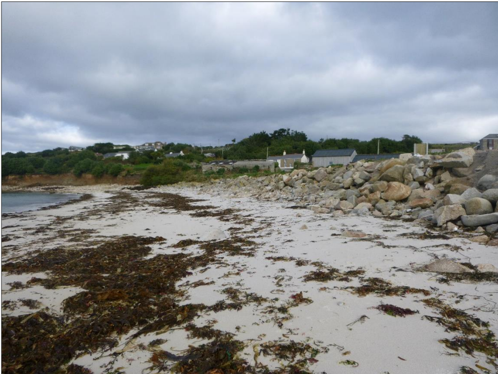
Figure 7: Looking north along the existing informal revetment where it interfaces with the existing dune defence.
