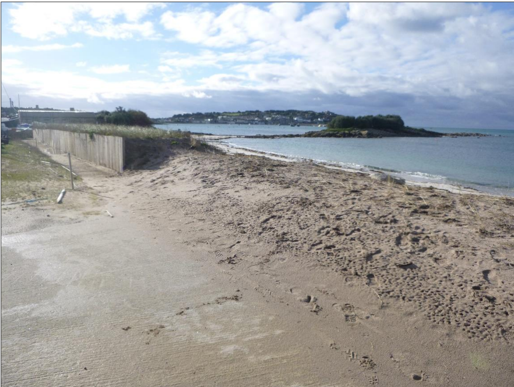
Figure 5: View of the existing dune defence and its timber sleeper construction. Note the low spot of the existing bank in the foreground that was formerly used as a temporary beach access point during the St. Mary's quay extension works in 2014/15.
