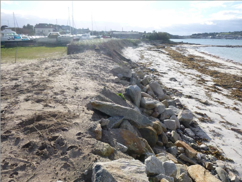
Figure 4: Looking south at the midpoint of the beach showing the interface between the existing dune defence in the background and the ad-hoc revetment in the foreground.
