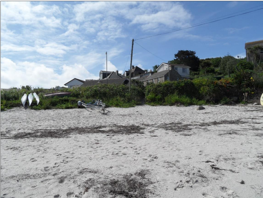
Figure 3: Southwest corner of Porth Mellon beach where the revetment is proposed. Note telegraph pole that may need to be relocated to accommodate the revetment.
