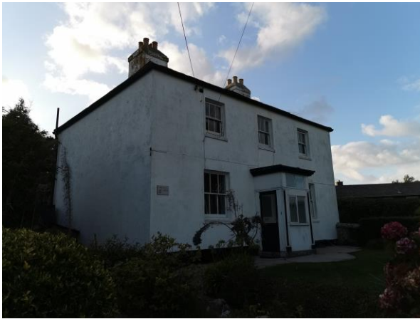
Photo 1. Showing the front of the house from the south east
