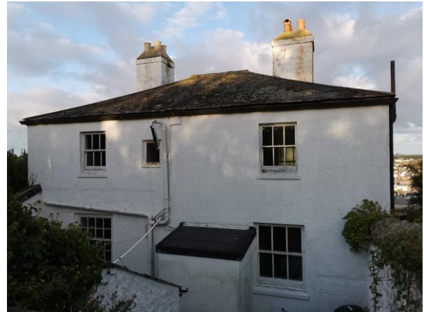
Photo 2. Showing the rear of the house from the west
